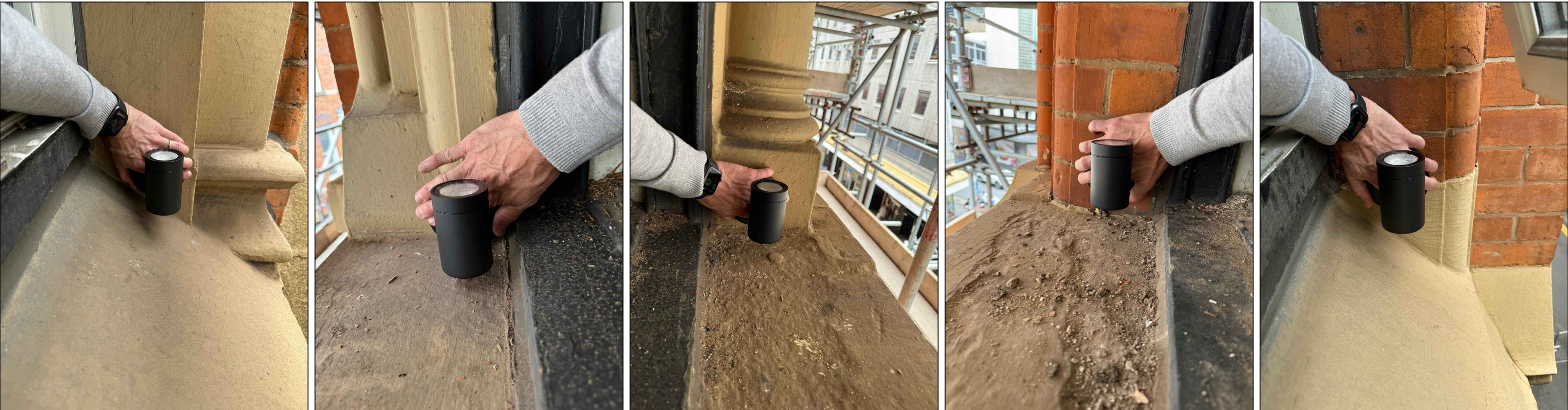
RAL 9005 FITTING WITH VARIOUS SECTIONS OF EXTERNAL MASONRY
