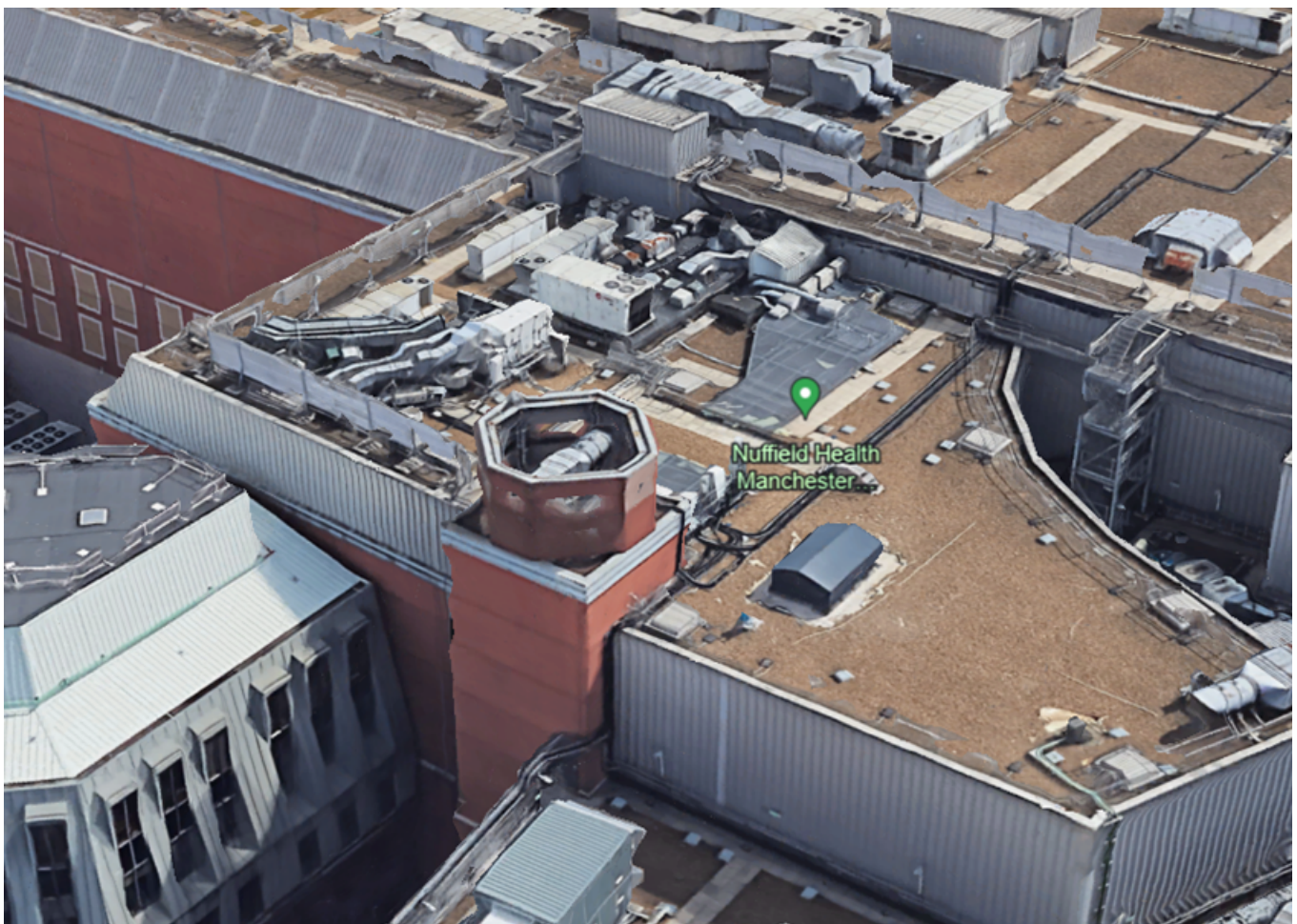
Existing Roof Plant Area
