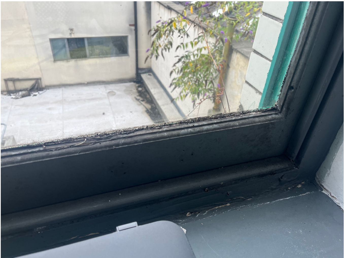
Condition of window frames on site (27 August 2024)
