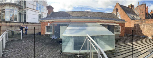
EXISTING CONDITIONS AT LOCATIONS FOR PLANT SCREEN.
