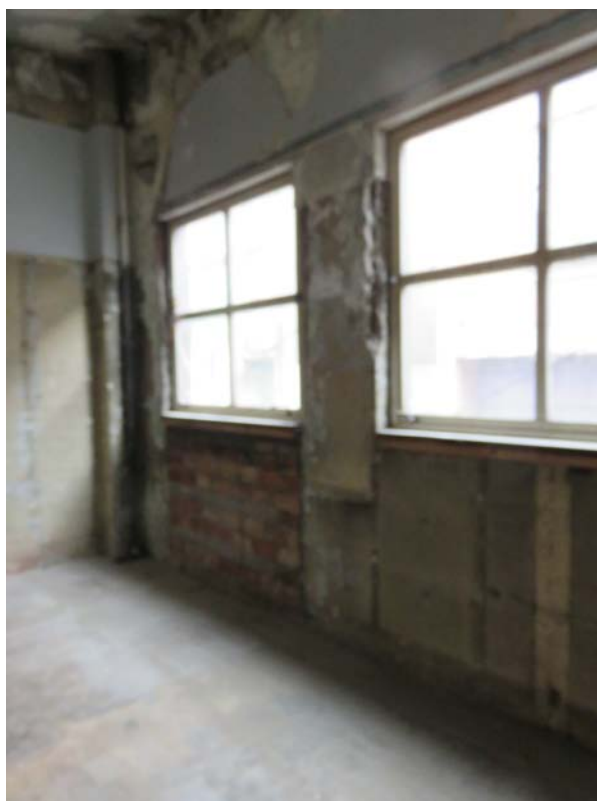
View looking at Richmond St from Ground floor.
