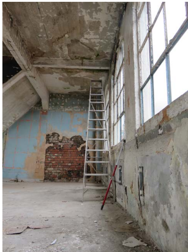
View looking to front windows from the top of the stairs on the 2 nd Floor.
