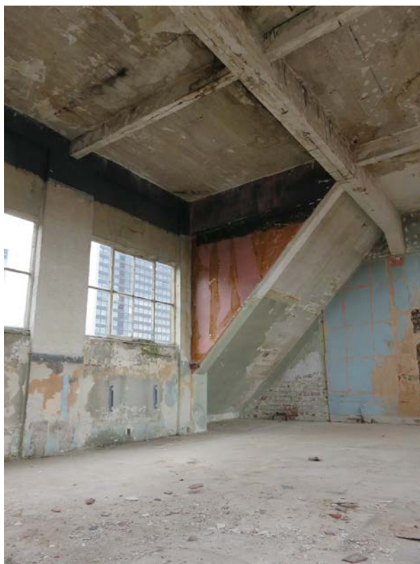
View looking to rear windows from the top of the stairs on the 2 nd Floor.
