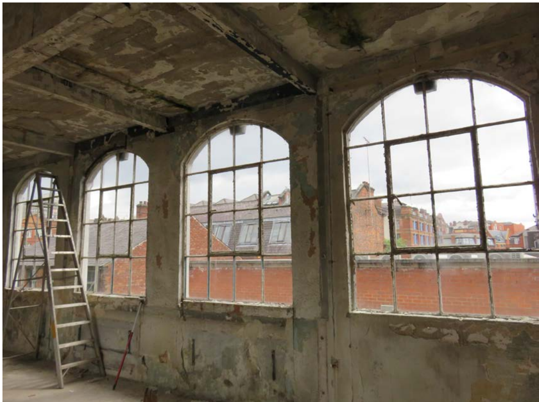
View looking at Richmond St from Ground floor.
