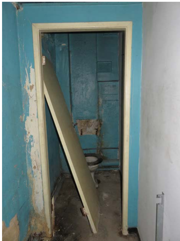
View of the existing toilets at the Basement.
