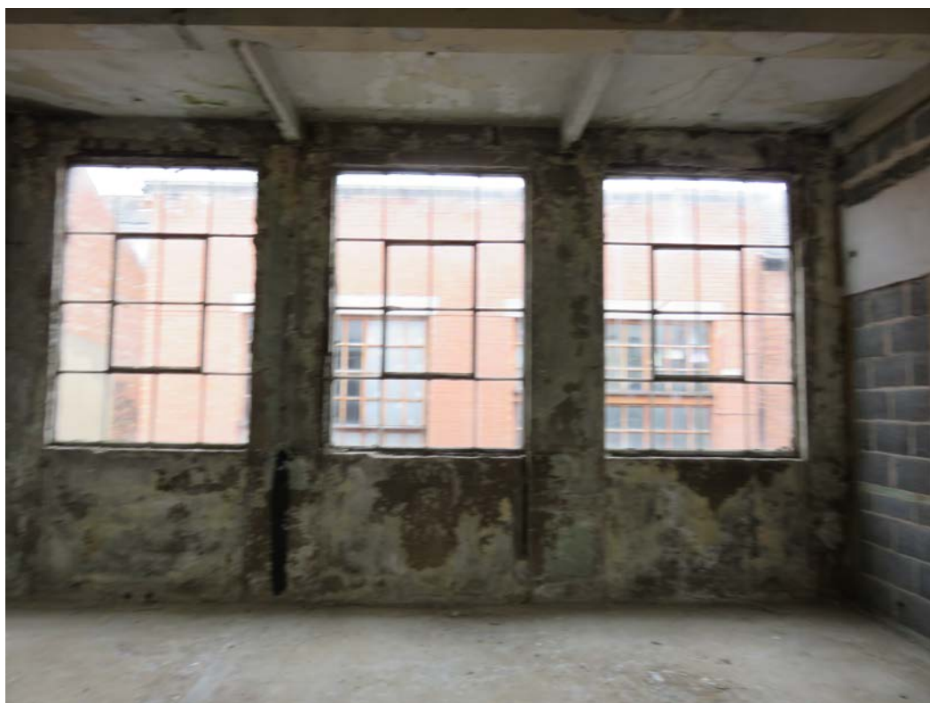
View of the windows in the front facade on 1 st Floor.
