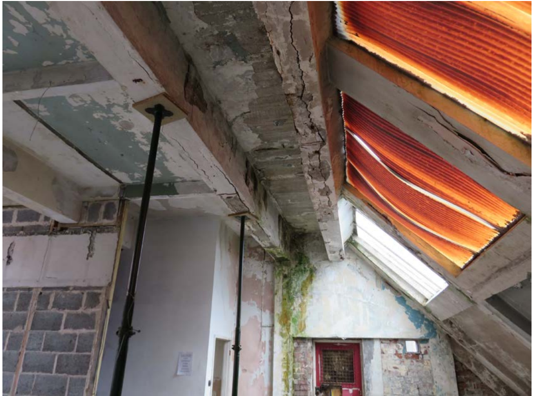
View of the concrete beam, windows and emergency door on the 1 st Floor.
