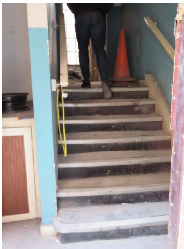
View of the stairs at the existing main entrance.
