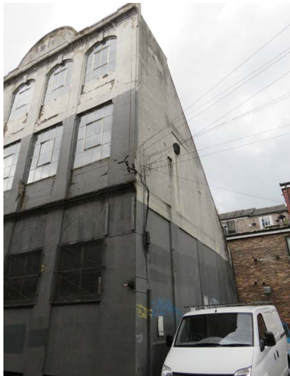
View showing from east side of Richmond St of the existing building.
