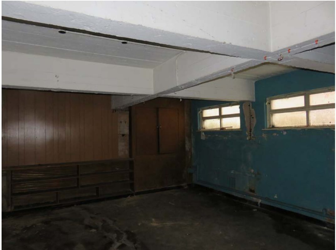
View of the front facade from Basement.
