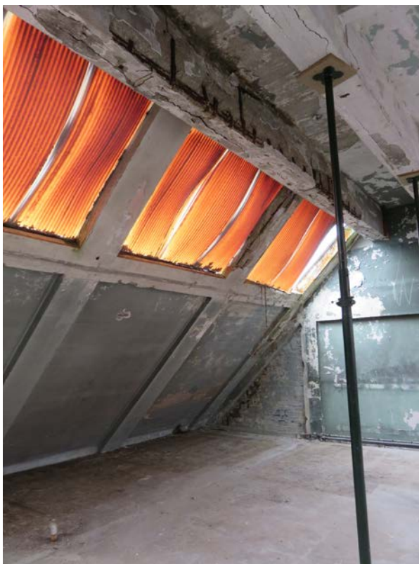
View of the rear pitched roof and windows on the 1 st Floor.
