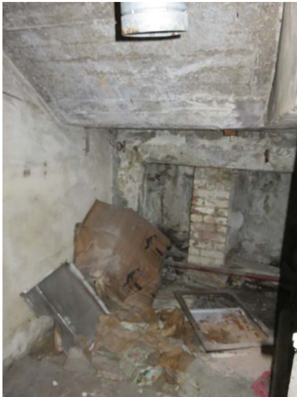
View of the bottom of the stair on the Basement.
