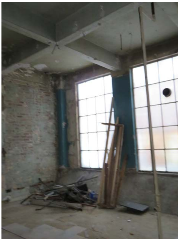
View of the windows to back alley on Ground floor.
