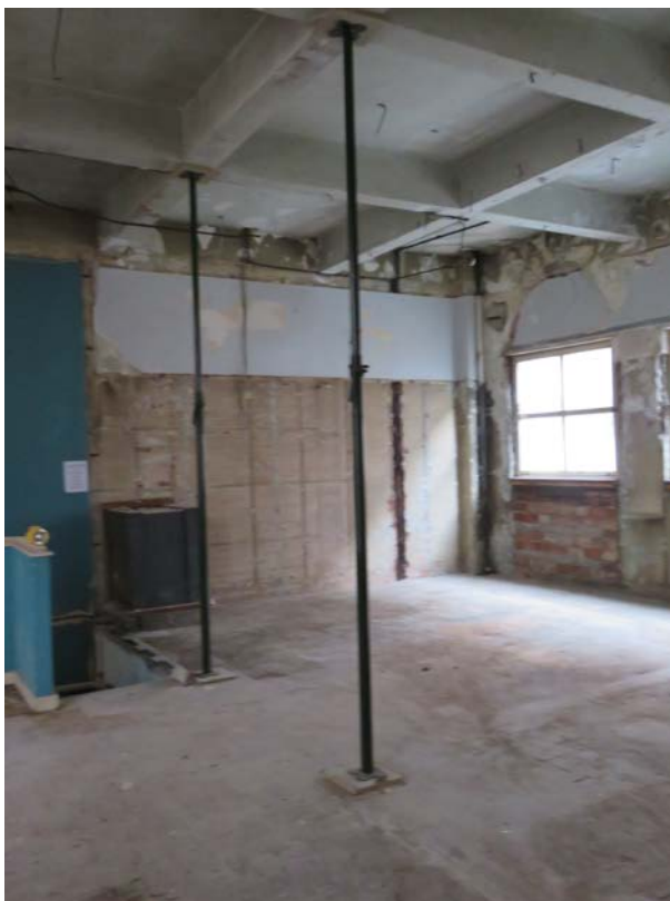
View of the main room and stair to basement at the Ground floor.
