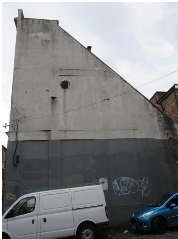
View of the East side elevation.
