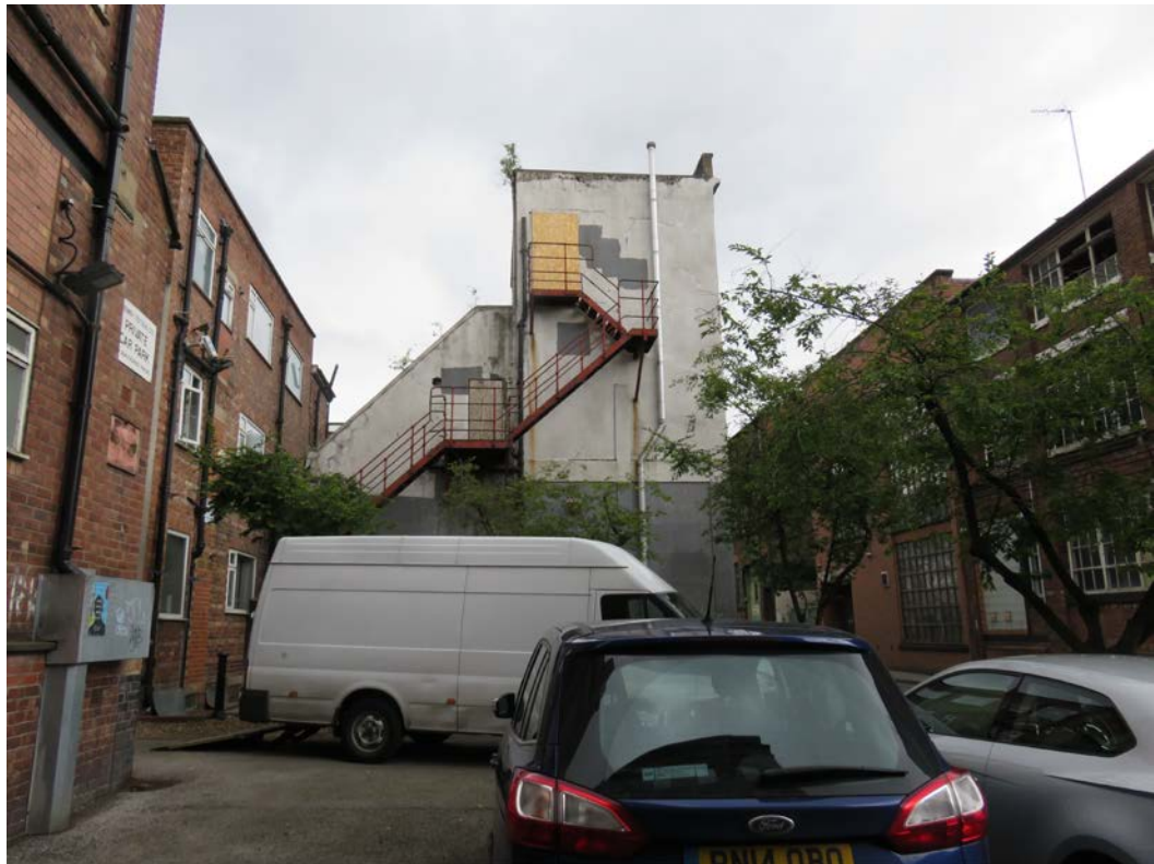
View of the East side elevation.
