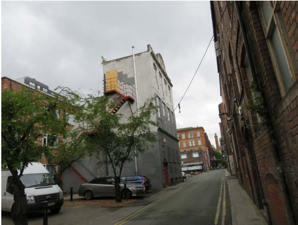
View showing from west side of Richmond St of the existing building.
