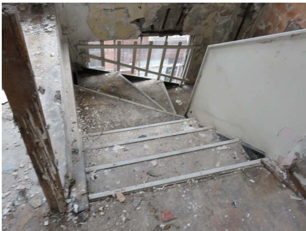
View looking at the landing of the stairs on the 2 nd Floor.
