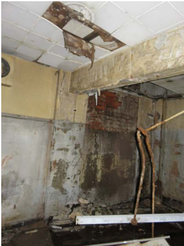
View of the back room on the Basement.
