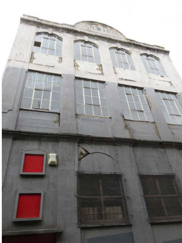
View looking to the front Facade.
