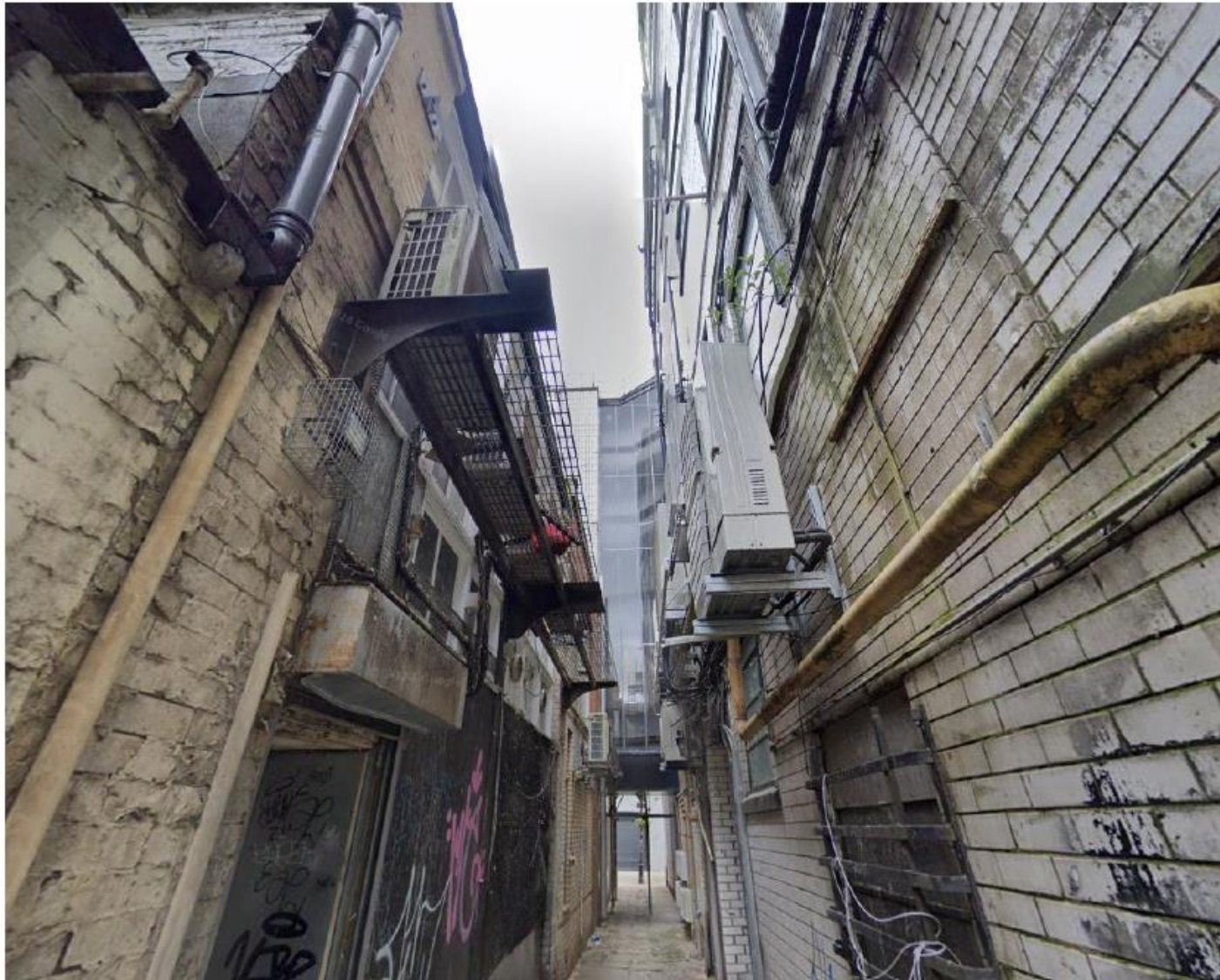
Location of Plant backing onto Mayo Street Alleyway
