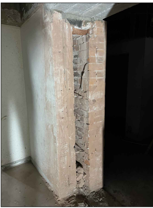
Opening 1- Existing Photo
