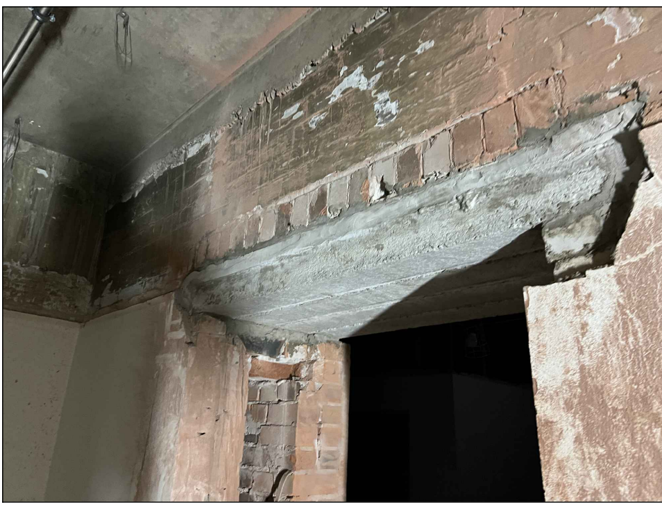
Opening 1- Existing Photo
