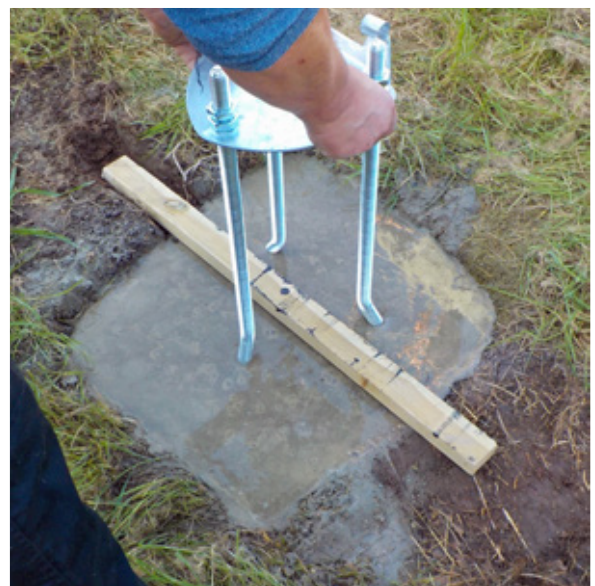
Insert the hinged base lower plate assembly. Check the direction of fall!
