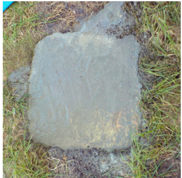
Poured, wet, concrete - move to next stage before it starts to dry!!
