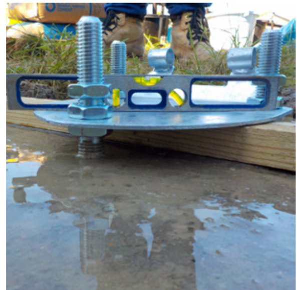
Once level allow concrete to fully set.
