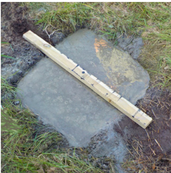
Use a piece of timber to help with levelling
