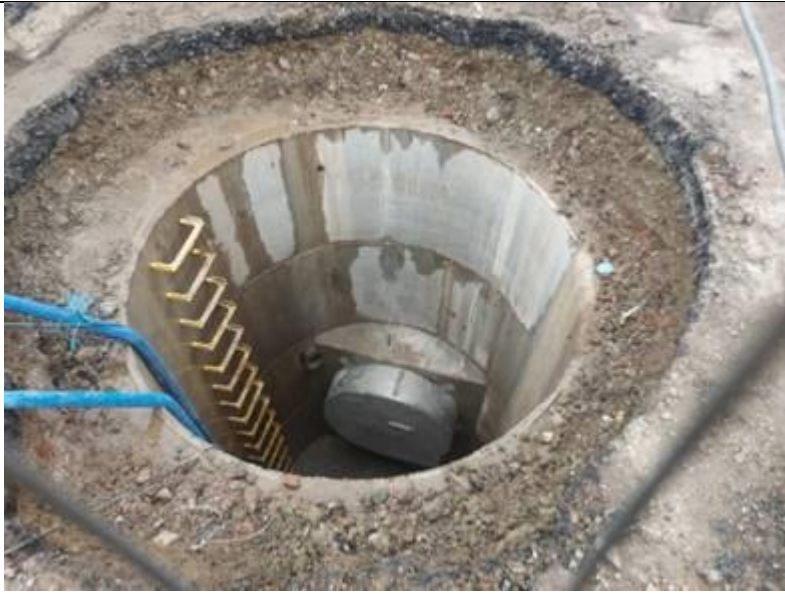
Picture 3 shows the installation of Vortex Flow Control within manhole reference SWMH157.
