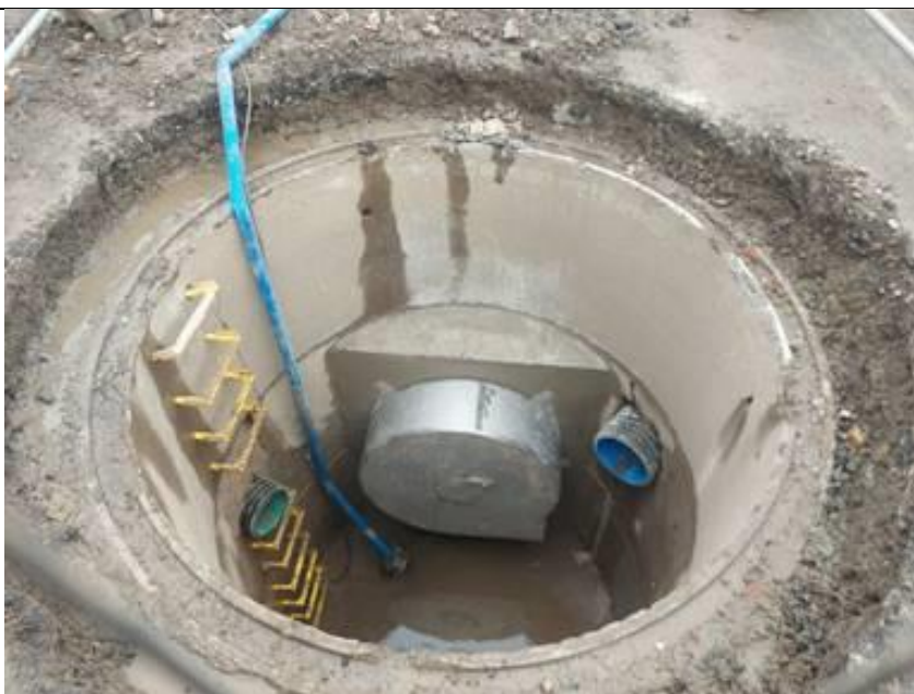
Picture 2 shows the installation of Vortex Flow Control within manhole reference SWMH138.
