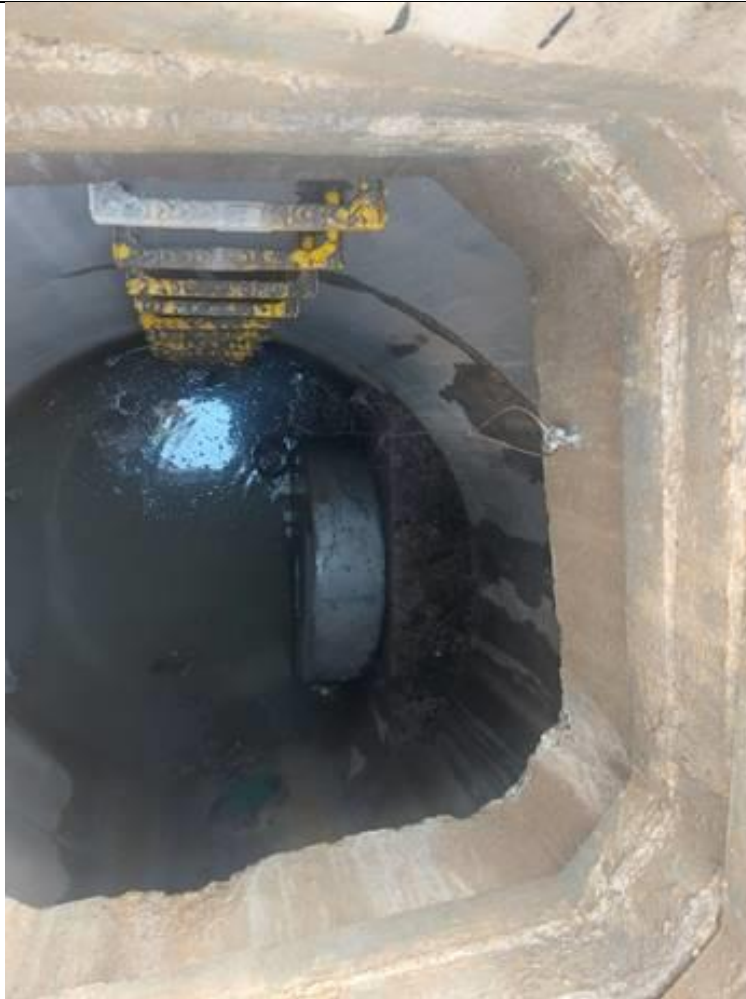
Picture 1 shows the installation of Vortex Flow Control within manhole reference SWMH153.
