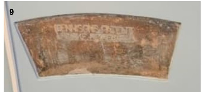
Exposed brick arch of a fireplace
