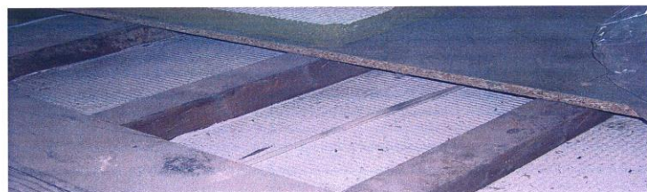
Figure 17 Karma TNF70 batts friction fitted between joists
