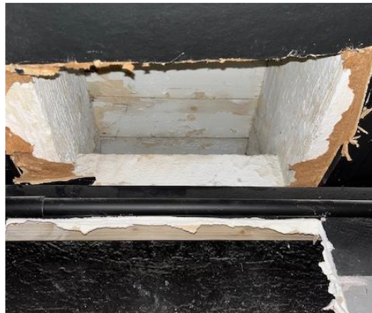
Figure 16 Ceiling of first floor
