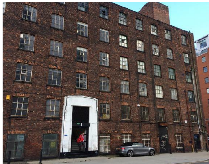
Figure 1 Street view of site
