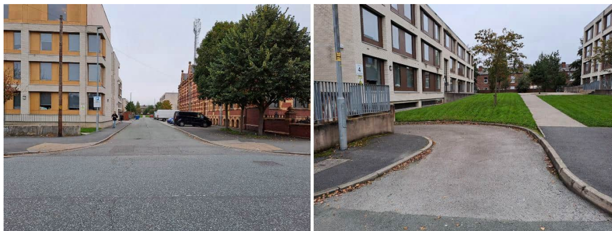
Figure I: Bax Road Access from Hathersage Road (left) and Access to Blocks 4 and 3 (right)
