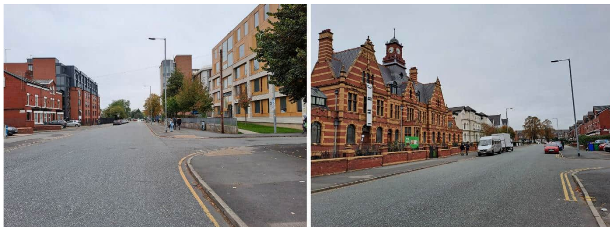
Figure K: Hathersage Road around the junction with Bax Road
