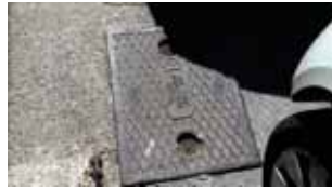
Photograph 4 (P4) View of man hole cover on site
