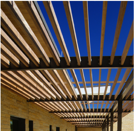
(above) Hardwood timber louvers to roof. Angled to obscure views from both the apartments above and elevated viewpoitns from the bridge approach
