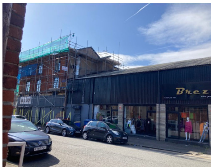
View of rear elevation
