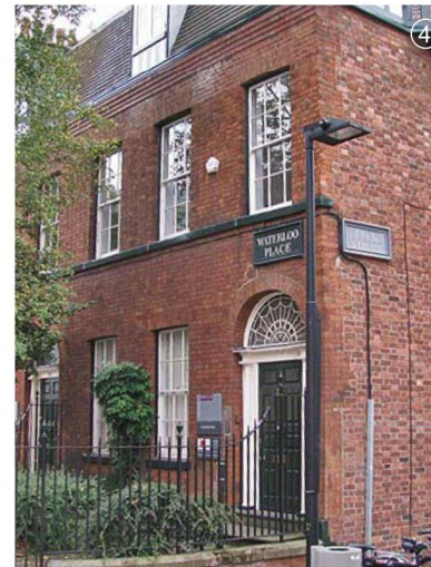
Semi circular fan light visible from Oxford Road
