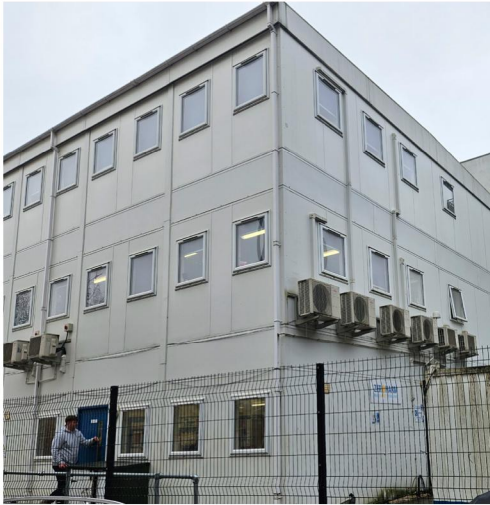
Existing Cabin's Exterior
