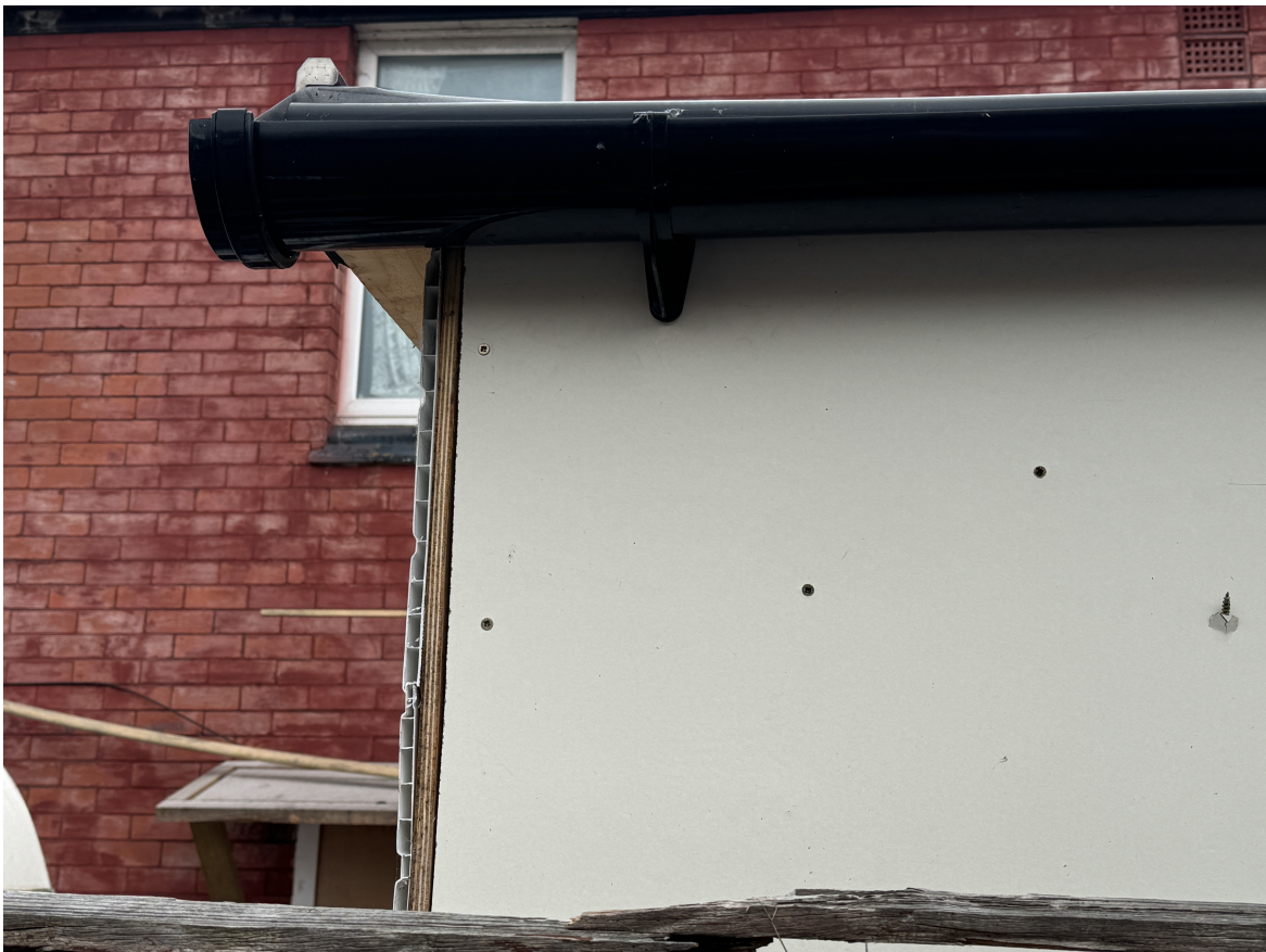
Figure 2. Finish of as built structure.
