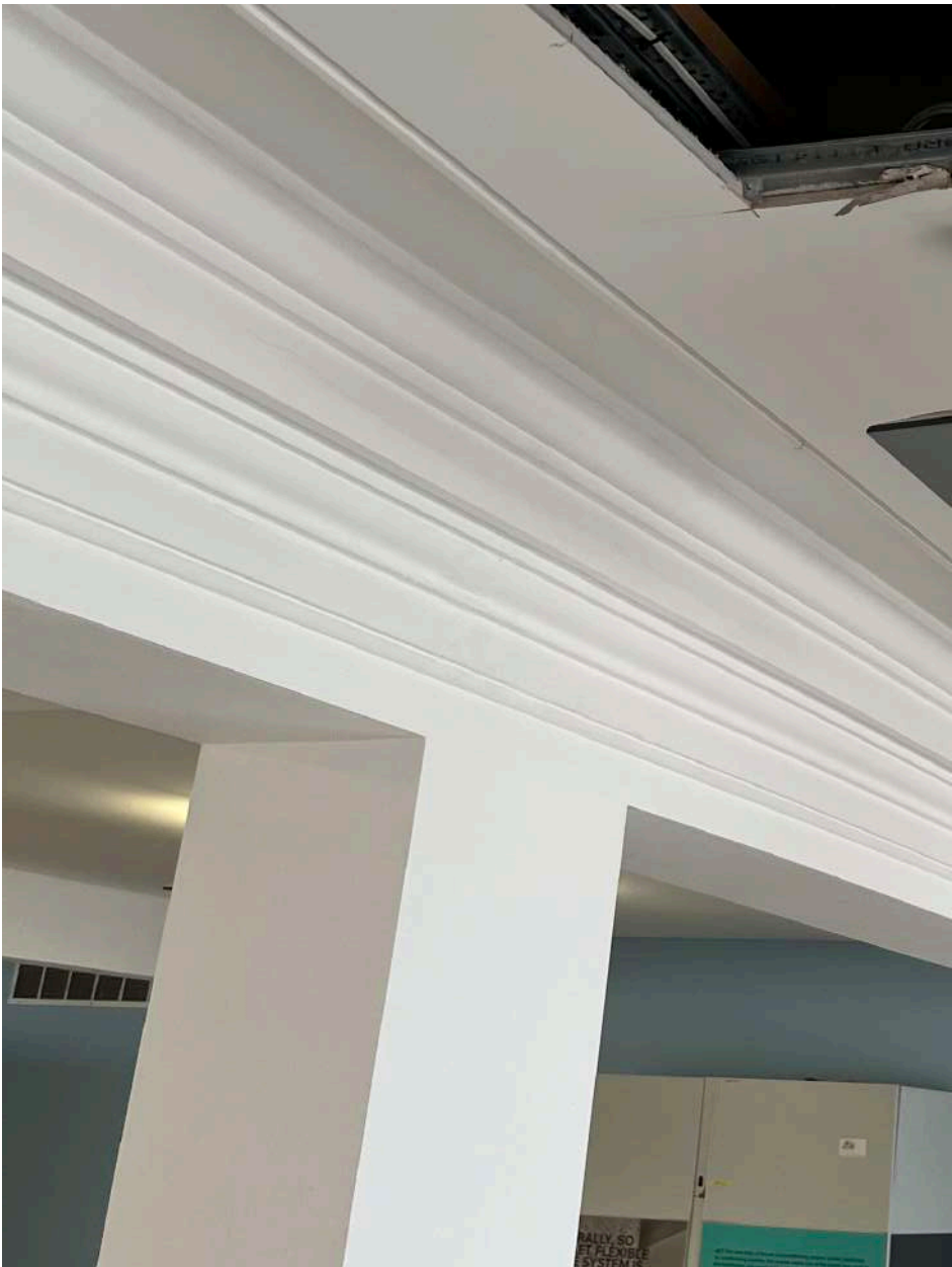
Typical Insitu Cornicing
