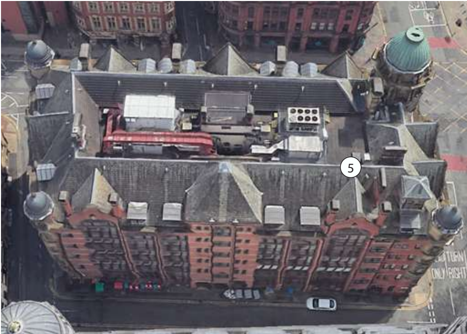
Aerial View - Roofscape
