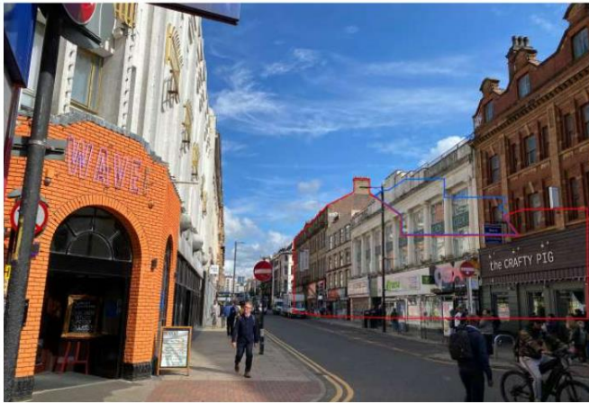
Figure 48 – View along Oldham Street towards the Hall. The adjacent buildings screen the new additions from view.
