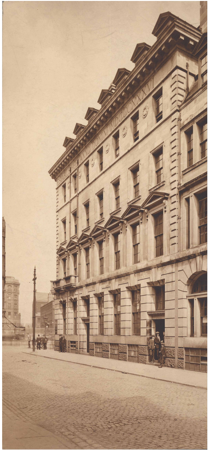
Archive photo reference of original facade
