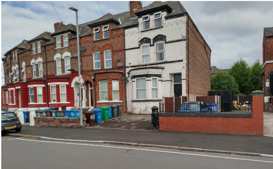
Ffg.1 – Application property viewed from Richmond Grove
