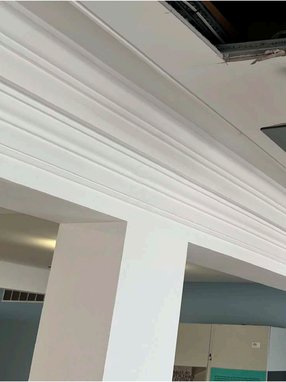
Typical Insitu Cornicing
