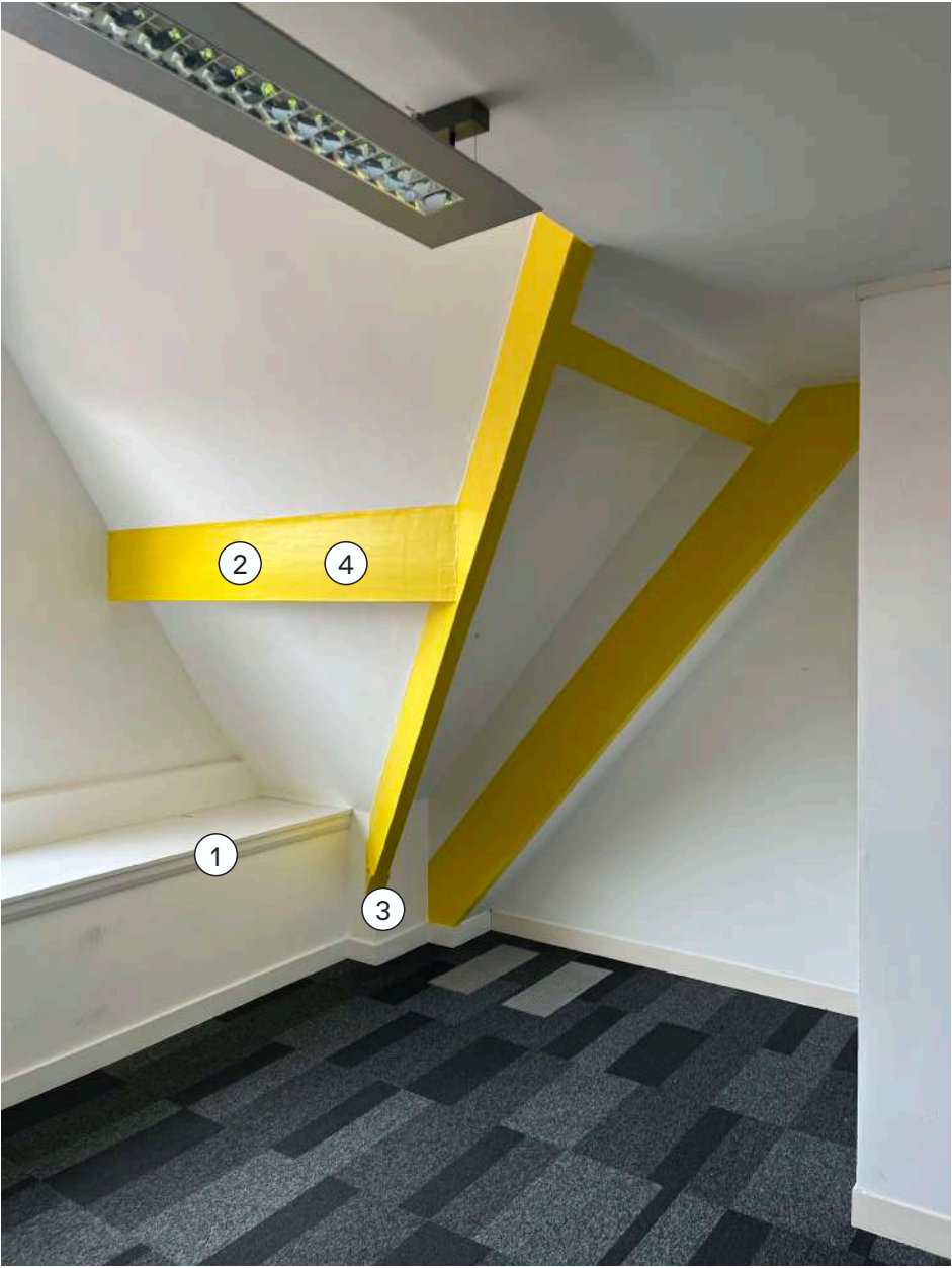
Typical Existing Raked Ceiling
