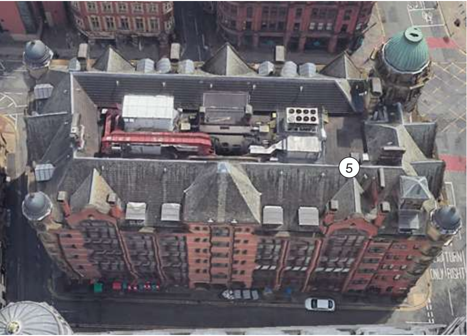
Aerial View - Roofscape
