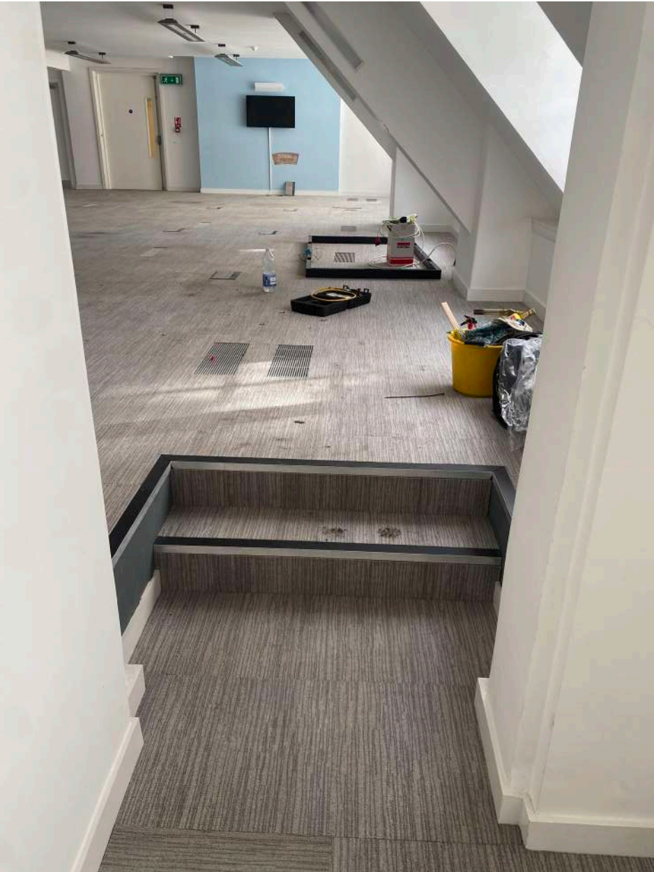
Typical Existing Level Change
