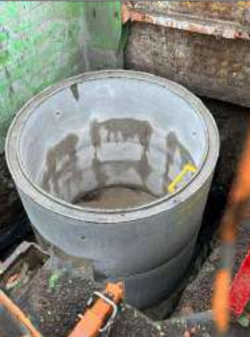
Pictures 9 & 10 shows the construction of the surface water demarcation manhole prior to the connection into the public sewer.
