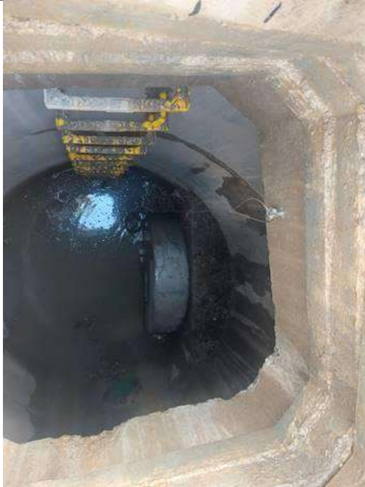
Picture 10 shows the installation of Vortex Flow Control within manhole reference SWMH153.
