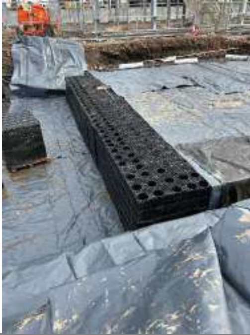
Pictures 7 & 8 shows the Attenuation Tank No 2 being constructed. The geocellular units are being laid over the impermeable membrane wrapped/sealed.
