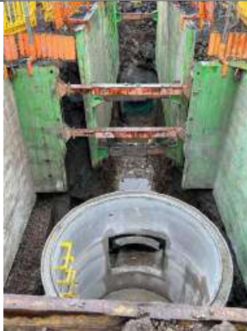
Pictures 9 & 10 shows the construction of the surface water demarcation manhole prior to the connection into the public sewer.
