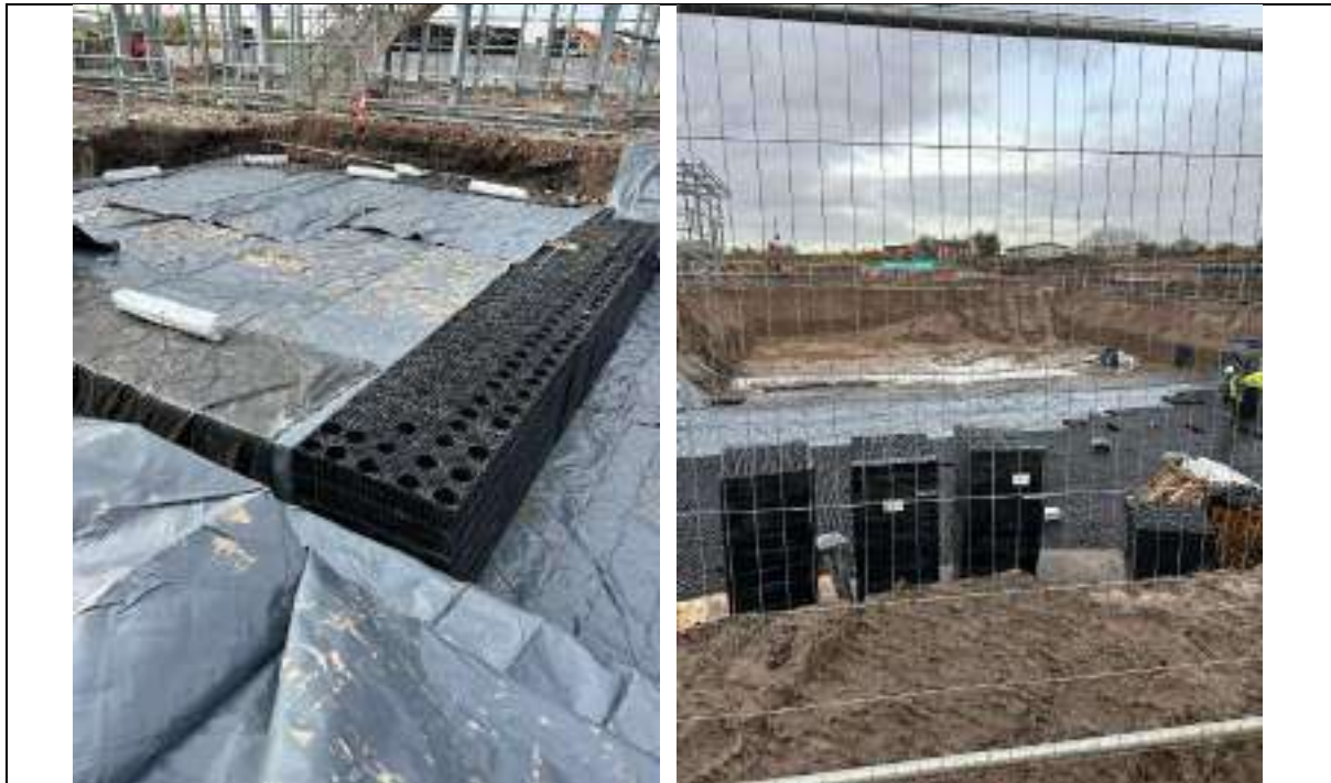
Picture 1 & 2 shows the installation of Attenuation Tank No 1.
