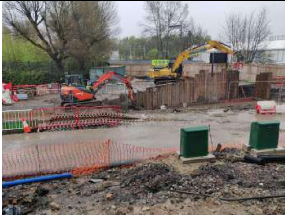
Picture 5 show the temporary excavation works for the oil separator installation.
