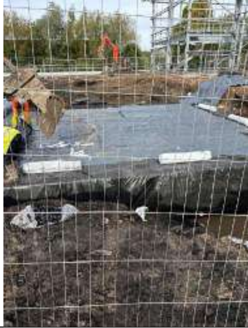
Pictures 7 & 8 shows the Attenuation Tank No 2 being constructed. The geocellular units are being laid over the impermeable membrane wrapped/sealed.
