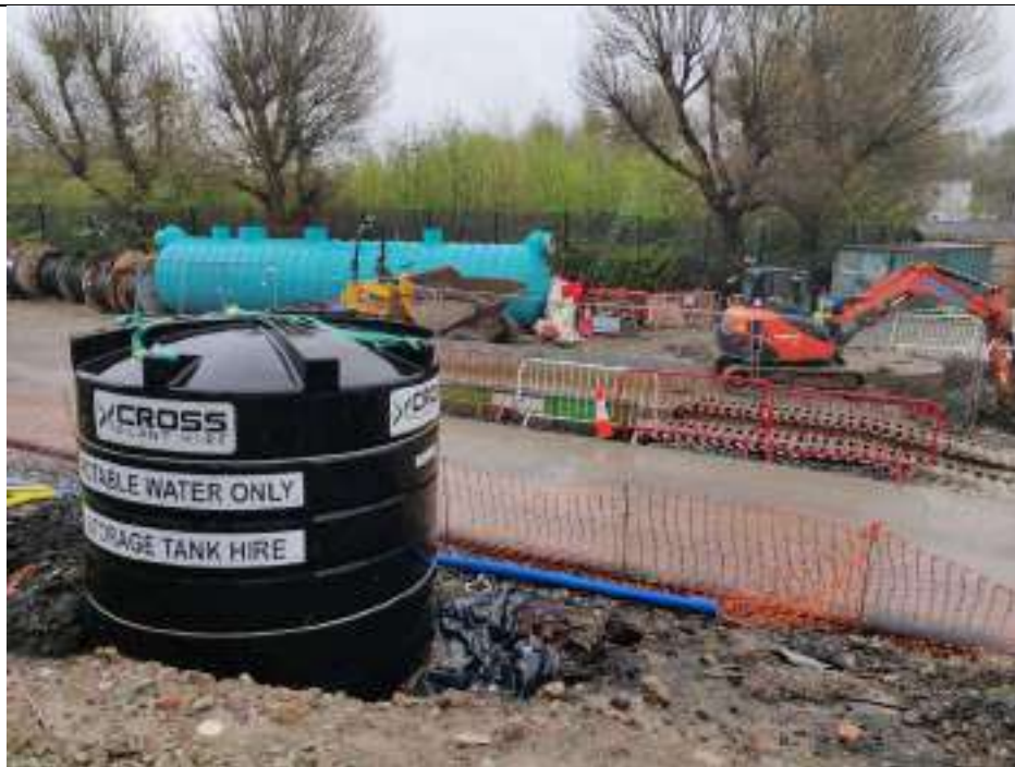
Picture 6 show the oil separator installation besides the temporary works excavation for its installation.
