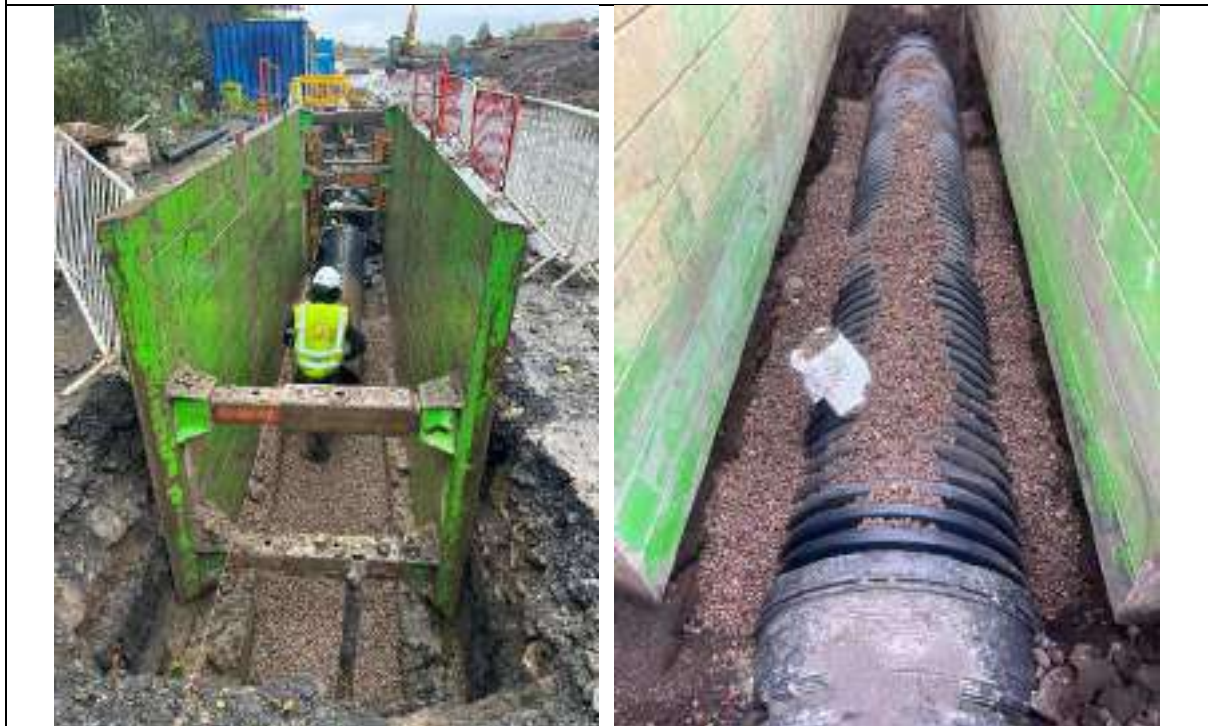
Pictures 3 & 4 shows the construction of the main surface water sewer laid along the access road.
