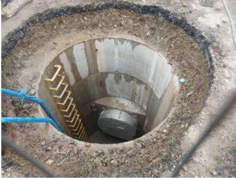
Picture 13 shows the installation of Vortex Flow Control within manhole reference SWMH157.
