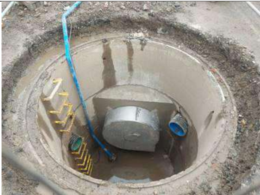
Picture 12 shows the installation of Vortex Flow Control within manhole reference SWMH138.
