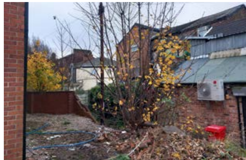
View to the rear of the existing block showing poor quality amenity space.
