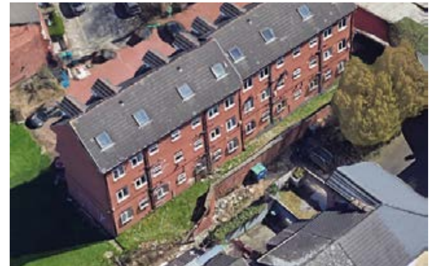
View to the rear of the existing block showing poor quality amenity space.
