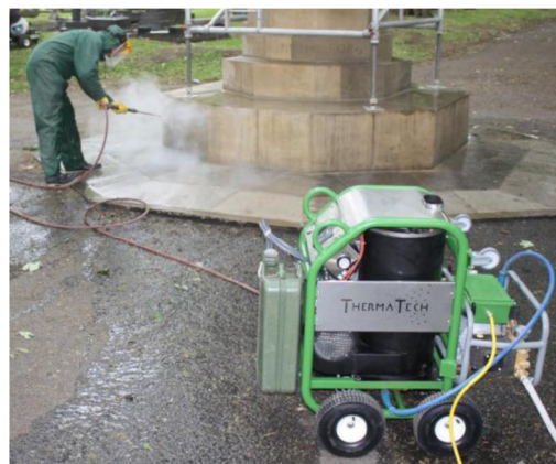
Fig 1. The ThermaTech system in use.
