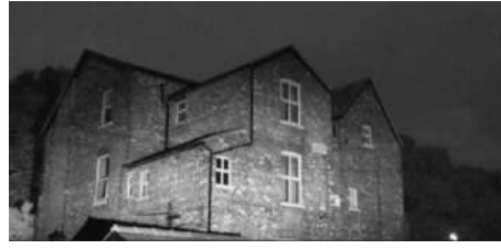
A3.10: Building B1; End of Survey
