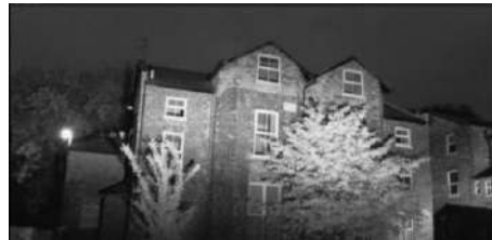
A3.12: Building B2; End of Survey
