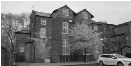
Plate A3.3: Building B2; Start of Survey
