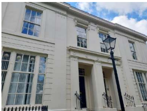
Plate 4.12: North Elevation; Painted and Found in Good Condition .
