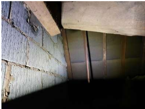
Plate 4.7: Area within The Attic Space, Separated By Breezeblocks
