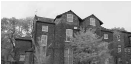
A3.11: Building B2; Start of Survey
