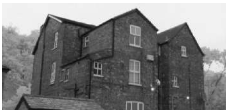
A3.5: Building B1; Start of Survey
