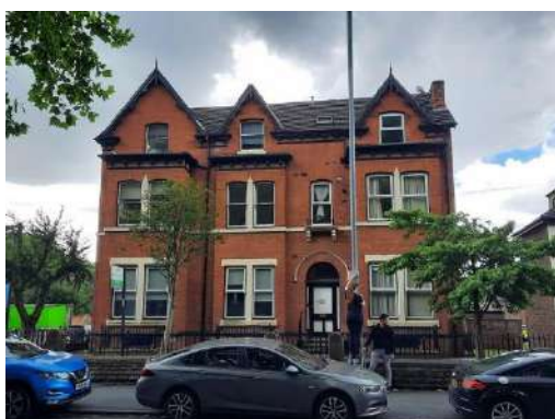
Plate 4.3: Ornate Fascia Boards on Southern Elevation
