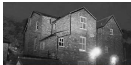
A3.6: Building B1; End of Survey
