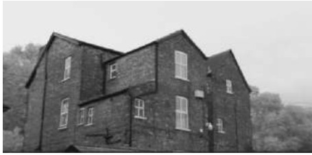
A3.9: Building B1; Start of Survey
