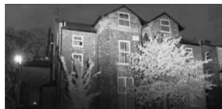
A3.8: Building B2; End of Survey
