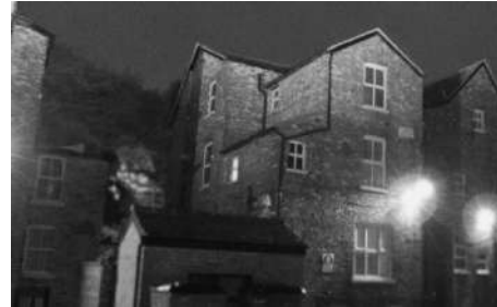
Plate A3.2: Building B1; End of survey.
