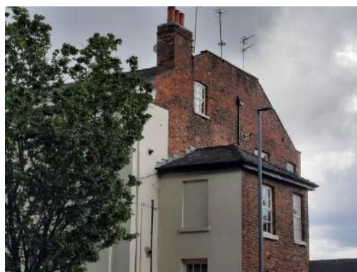
Plate 4.11: Mansard Style Roof, Wooden Fascia Boards, and Wooden Framed Windows Consistent Throughout The Building.
