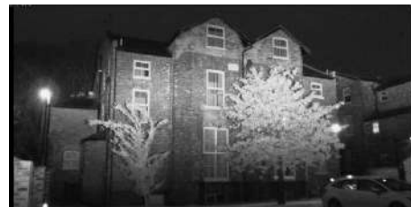
Plate A3.4: Building B2; End of Survey
