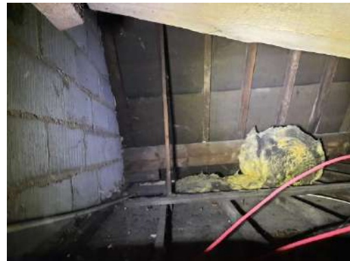
Plate 4.8: Some Areas of Insulation within the Roof Space
