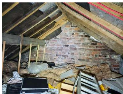
Plate 4.16: Inside of the Attic Space with Insulation and Aerial Cables Visible.
