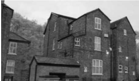
Plate A3.1: Building B1; Start of survey.
