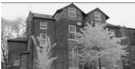
A3.7: Building B2, Start of Survey
