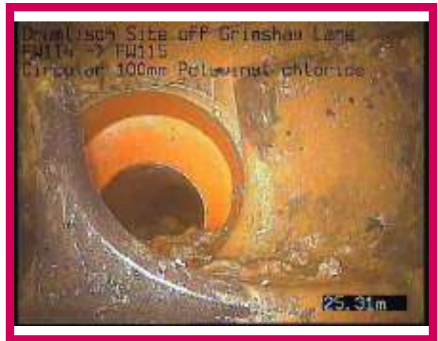
2, 00:02:09, 25.31 m Finish node, manhole, reference: FW115
