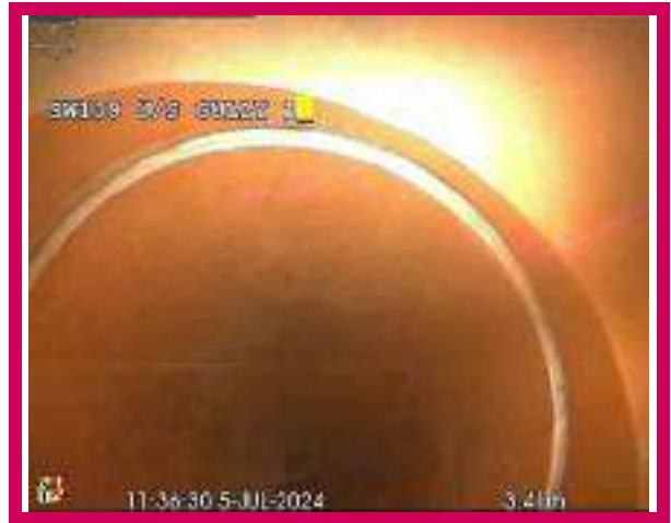
2, 00:00:25, 3.41 m Finish node, other special chamber, reference: Gully 1, Line reduces to 100mm before gully.
