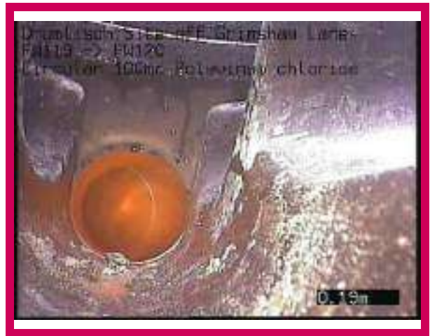
2, 00:00:36, 0.19 m Finish node, manhole, reference: FW120
