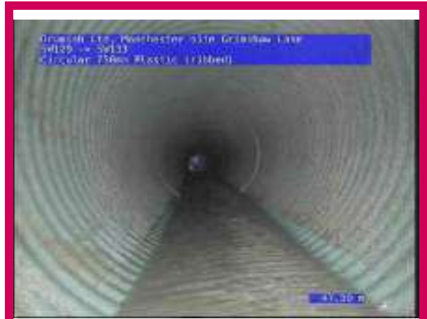
2, 00:04:00, 47.50 m Finish node, manhole, reference: SW133
