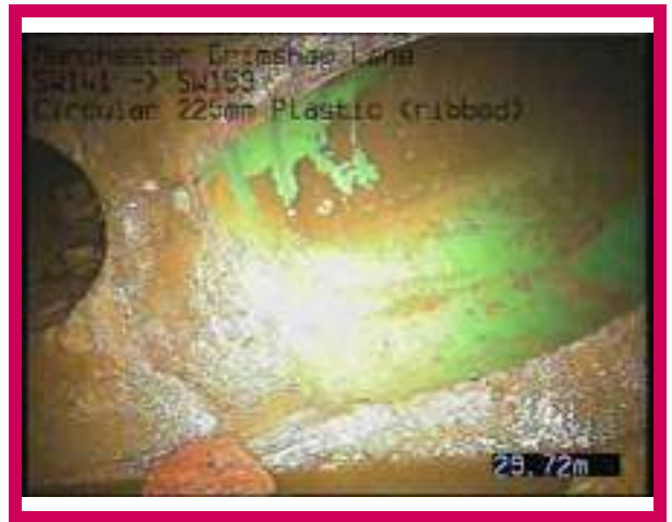
2, 00:02:28, 29.72 m Finish node, manhole, reference: SW153
