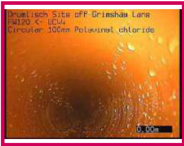
1, 00:00:00, 0.00 m Start node, manhole, reference: FW120
