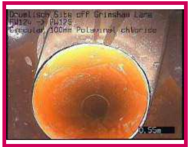
2, 00:00:53, 0.55 m Finish node, manhole, reference: FW125
