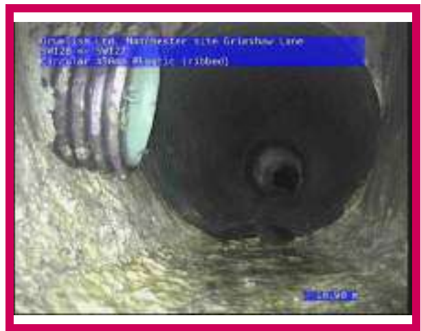
2, 00:00:44, 10.90 m Finish node, manhole, reference: SW127
