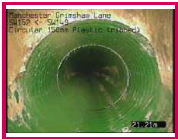
2, 00:02:46, 21.21 m Finish node, manhole, reference: SW149
