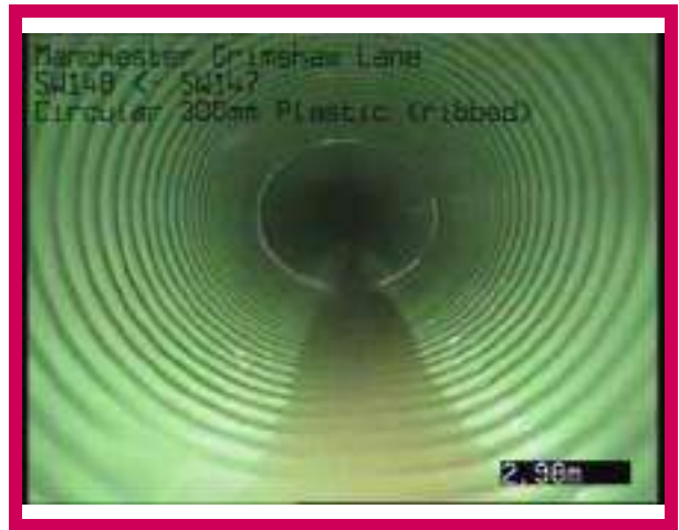
2, 00:01:53, 27.46 m Finish node, manhole, reference: SW147
