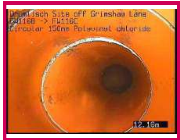
2, 00:01:40, 12.17 m Finish node, manhole, reference: FW116C, In View
