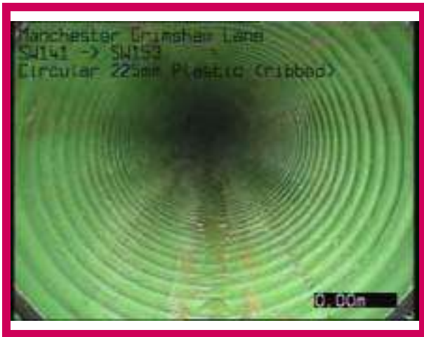
1, 00:00:00, 0.00 m Start node, manhole, reference: SW141
