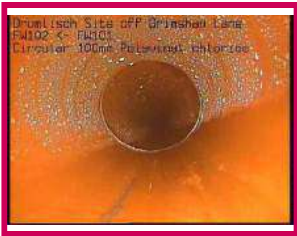
1, 00:00:00, 0.00 m Start node, manhole, reference: FW102
