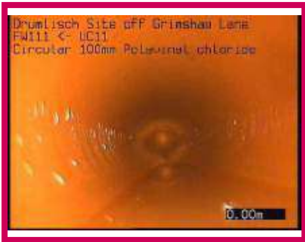
1, 00:00:00, 0.00 m Start node, manhole, reference: FW111
