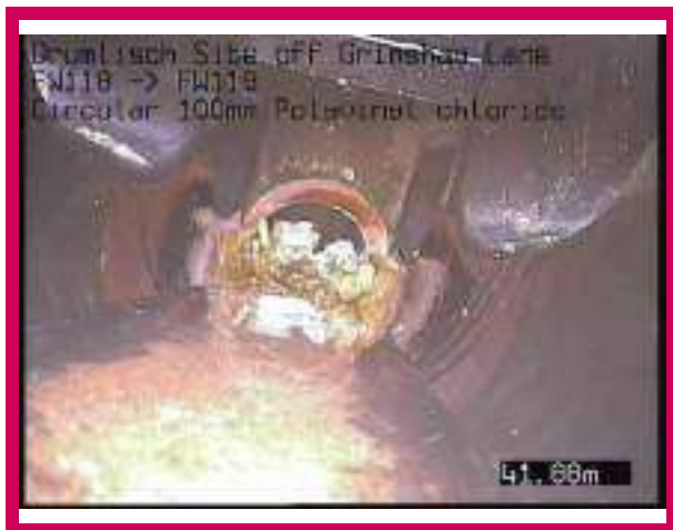
3, 00:03:04, 41.88 m Finish node, manhole, reference: FW119
