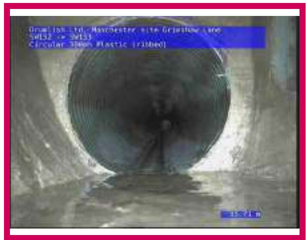
2, 00:02:41, 35.71 m Finish node, manhole, reference: SW153
