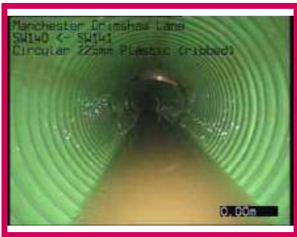
1, 00:00:00, 0.00 m Start node, manhole, reference: SW140
