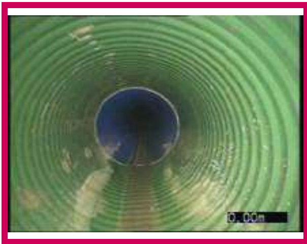
1, 00:00:00, 0.00 m Start node, manhole, reference: SW 125
