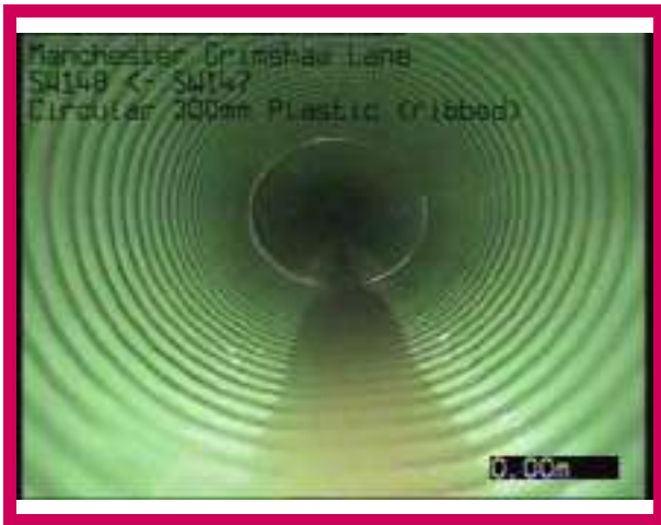
1, 00:00:00, 0.00 m Start node, manhole, reference: SW148
