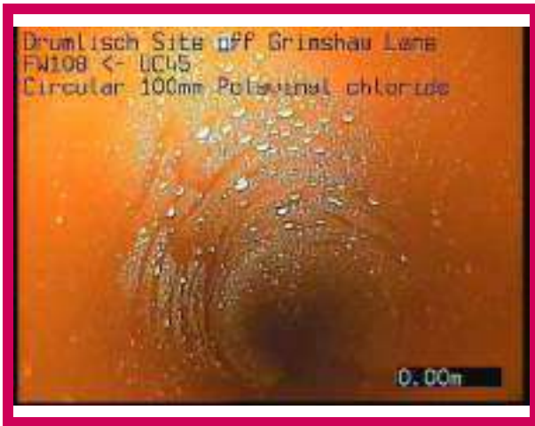
1, 00:00:00, 0.00 m Start node, manhole, reference: FW108
