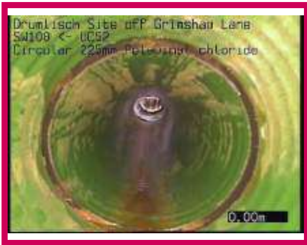
1, 00:00:00, 0.00 m Start node, manhole, reference: SW108
