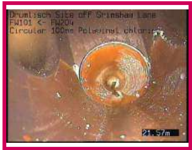
2, 00:01:30, 21.57 m Finish node, manhole, reference: FW204
