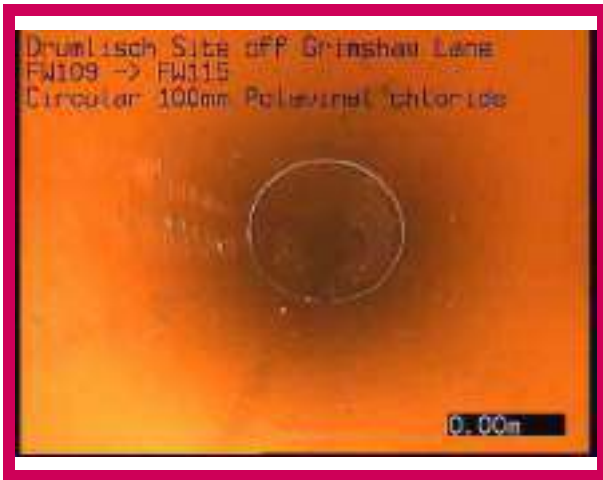
1, 00:00:00, 0.00 m Start node, manhole, reference: FW109
