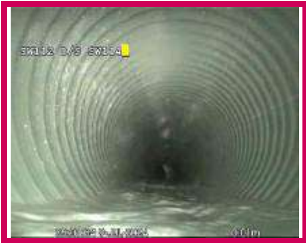
1, 00:00:00, 0.00 m Start node, manhole, reference: SW112
