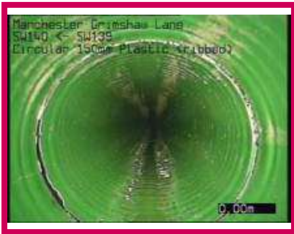
1, 00:00:00, 0.00 m Start node, manhole, reference: SW140
