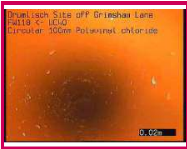
1, 00:00:00, 0.00 m Start node, manhole, reference: FW118
