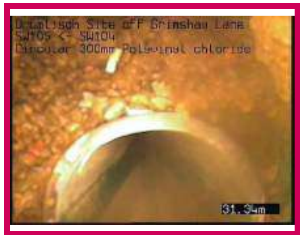
2, 00:07:04, 31.34 m Finish node, manhole, reference: SW104
