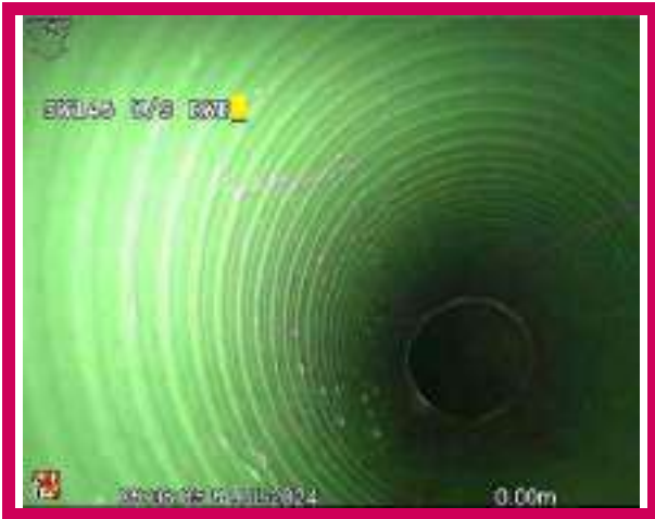
1, 00:00:00, 0.00 m Start node, manhole, reference: SW145
