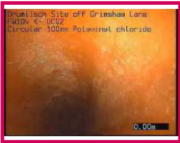
1, 00:00:00, 0.00 m Start node, manhole, reference: FW104
