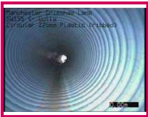
1, 00:00:00, 0.00 m Start node, manhole, reference: SW155
