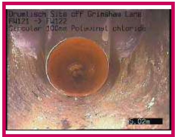
2, 00:00:32, 5.02 m Finish node, manhole, reference: FW122
