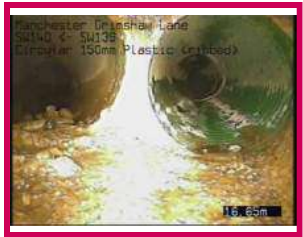
2, 00:02:37, 16.65 m Finish node, manhole, reference: SW139
