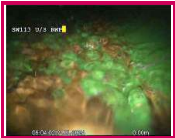
1, 00:00:00, 0.00 m Start node, manhole, reference: SW113
