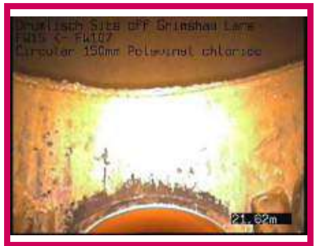
2, 00:02:33, 21.62 m Finish node, manhole, reference: FW107
