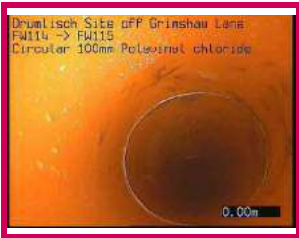
1, 00:00:00, 0.00 m Start node, manhole, reference: FW114
