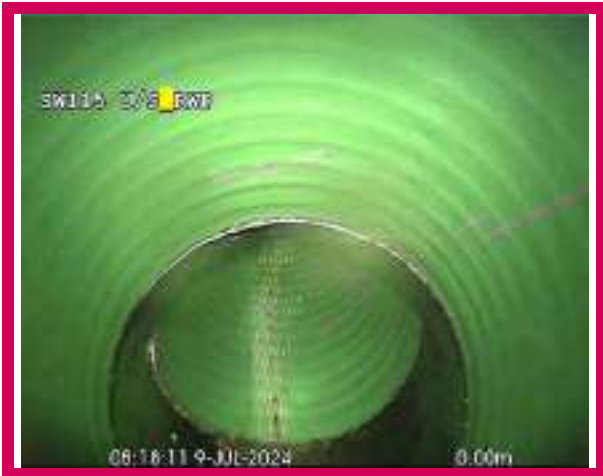
1, 00:00:00, 0.00 m Start node, manhole, reference: SW115
