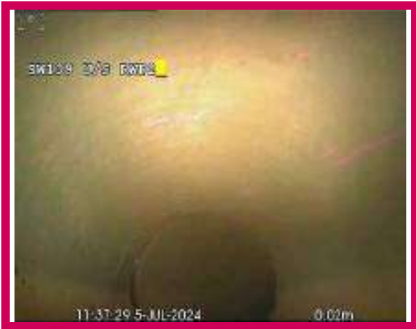
1, 00:00:00, 0.00 m Start node, manhole, reference: SW139
