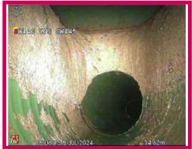
2, 00:00:34, 14.62 m Finish node, manhole, reference: SW145
