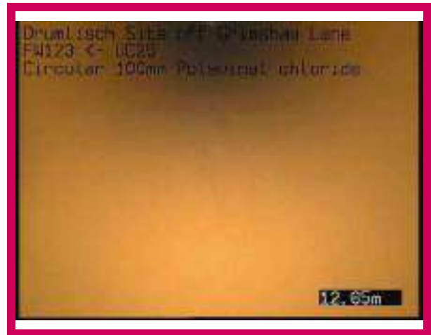
2, 00:01:09, 12.65 m Finish node, other special chamber, reference: UC25, In View unable to push round bends
