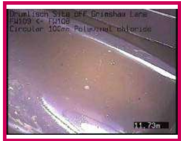
2, 00:00:53, 11.73 m Finish node, manhole, reference: FW108
