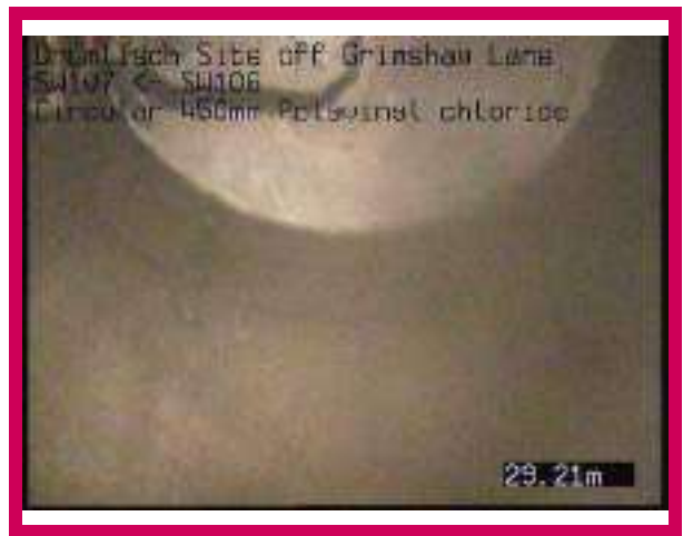
2, 00:02:48, 29.21 m Finish node, manhole, reference: SW106
