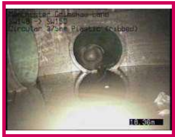
2, 00:01:39, 18.36 m Finish node, manhole, reference: SW150, MH is in a tank.
