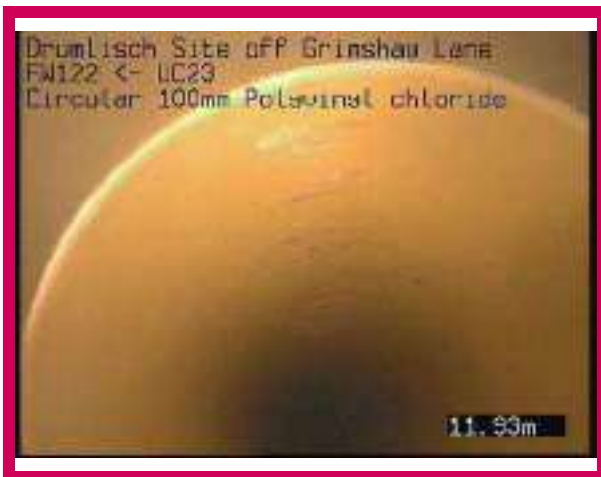
3, 00:01:30, 11.93 m Finish node, other special chamber, reference: UC23, In View
