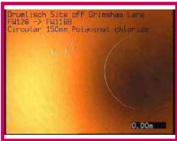
1, 00:00:00, 0.00 m Start node, manhole, reference: FW126
