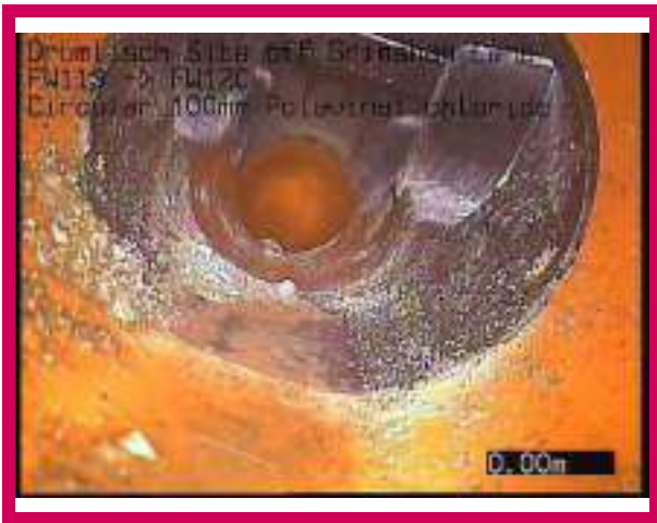
1, 00:00:00, 0.00 m Start node, manhole, reference: FW119
