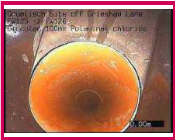
1, 00:00:00, 0.00 m Start node, manhole, reference: FW125
