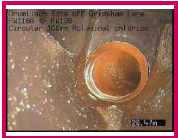
2, 00:01:26, 26.47 m Finish node, manhole, reference: FW128
