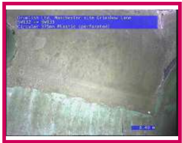
2, 00:00:37, 8.40 m Finish node, manhole, reference: SW133
