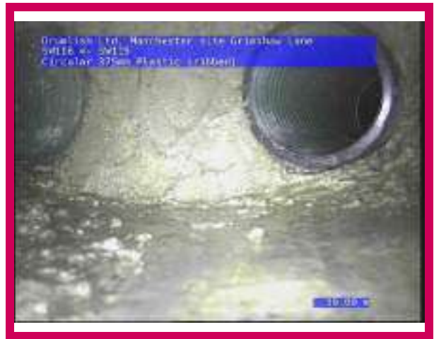
2, 00:02:11, 39.09 m Finish node, manhole, reference: SW115
