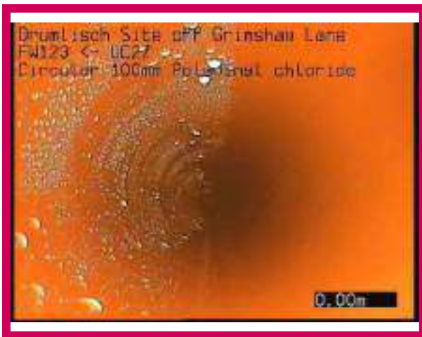
1, 00:00:00, 0.00 m Start node, manhole, reference: FW123
