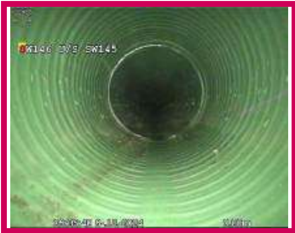
1, 00:00:00, 0.00 m Start node, manhole, reference: SW146
