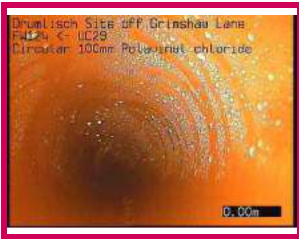
1, 00:00:00, 0.00 m Start node, manhole, reference: FW124
