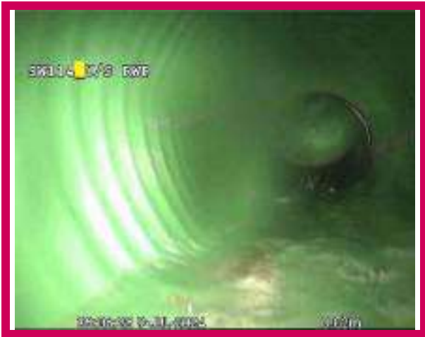
1, 00:00:00, 0.00 m Start node, manhole, reference: SW114
