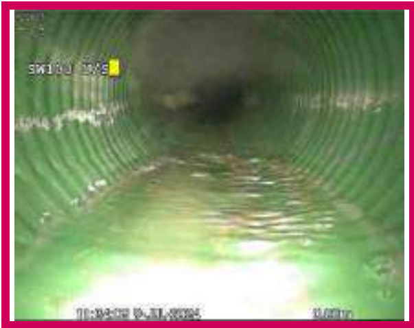
1, 00:00:00, 0.00 m Start node, manhole, reference: SW103
