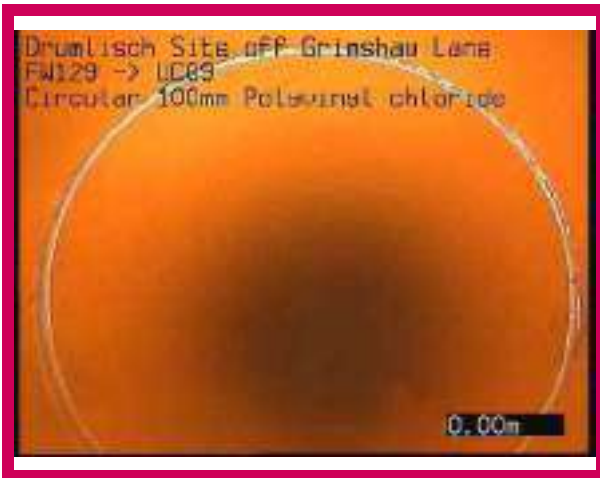
1, 00:00:00, 0.00 m Start node, manhole, reference: FW129
