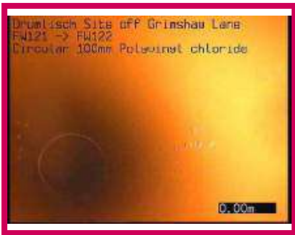
1, 00:00:00, 0.00 m Start node, manhole, reference: FW121
