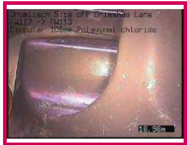
2, 00:01:09, 16.96 m Finish node, manhole, reference: FW113
