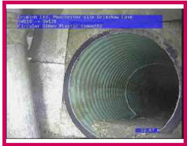
2, 00:00:58, 12.07 m Finish node, catchpit, reference: SW129
