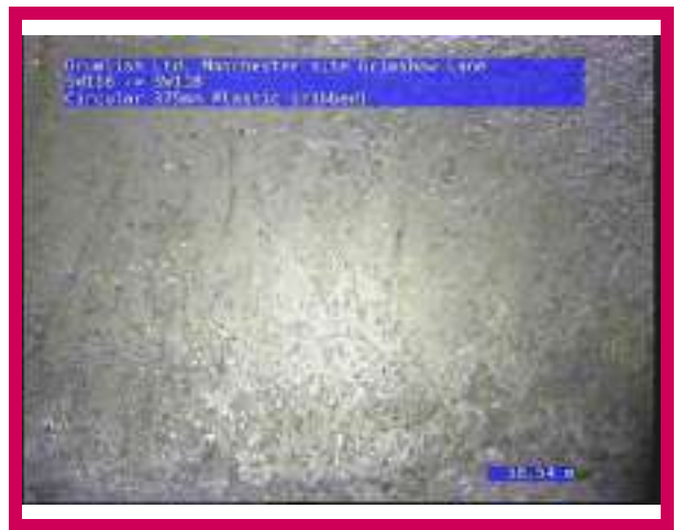
2, 00:01:57, 38.54 m Finish node, manhole, reference: SW118
