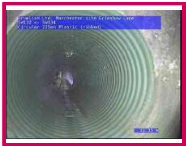
2, 00:02:03, 32.35 m Finish node, manhole, reference: SW134
