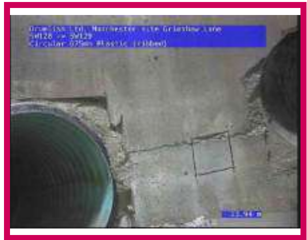
2, 00:00:51, 13.94 m Finish node, catchpit, reference: SW129
