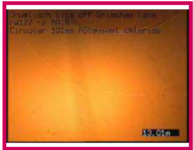
2, 00:01:13, 13.01 m Finish node, major connection without manhole, reference: MAIN
