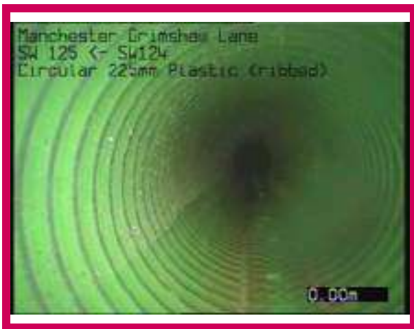
1, 00:00:00, 0.00 m Start node, manhole, reference: SW 125
