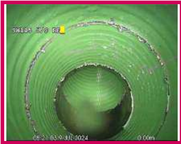
1, 00:00:00, 0.00 m Start node, manhole, reference: SW115
