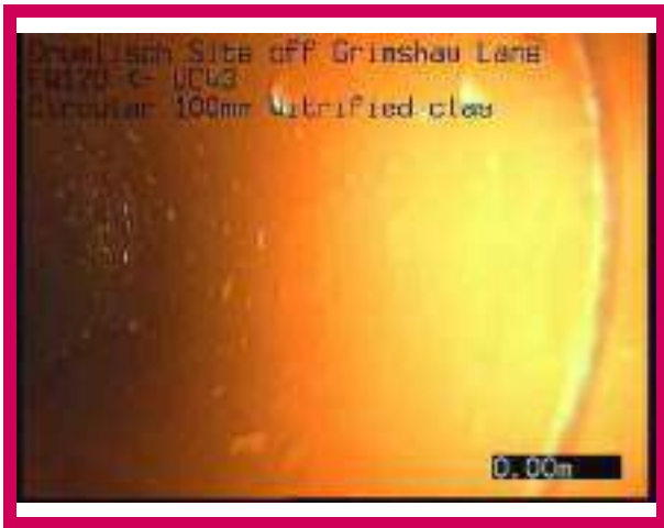
1, 00:00:00, 0.00 m Start node, manhole, reference: FW120
