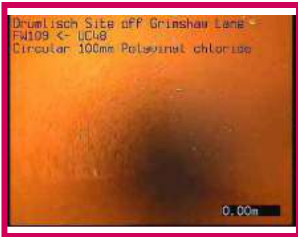
1, 00:00:00, 0.00 m Start node, manhole, reference: FW109
