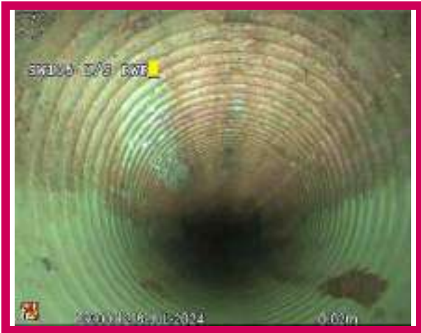
1, 00:00:00, 0.00 m Start node, manhole, reference: SW135
