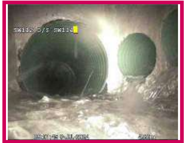
2, 00:00:10, 4.60 m Finish node, manhole, reference: SW114
