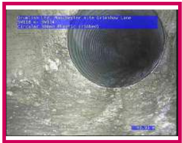
2, 00:02:13, 45.91 m Finish node, manhole, reference: SW114
