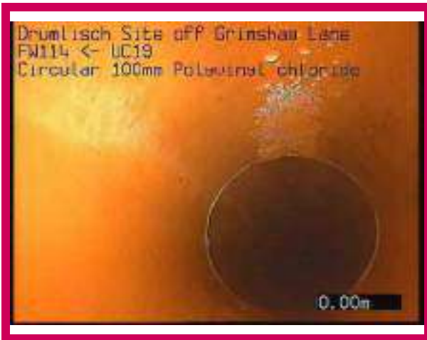
1, 00:00:00, 0.00 m Start node, manhole, reference: FW114
