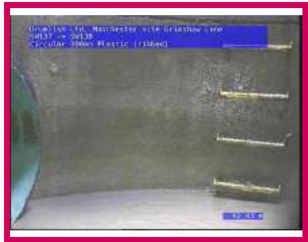
2, 00:02:21, 42.43 m Finish node, catchpit, reference: SW138
