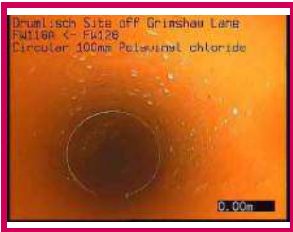
1, 00:00:00, 0.00 m Start node, manhole, reference: FW116A
