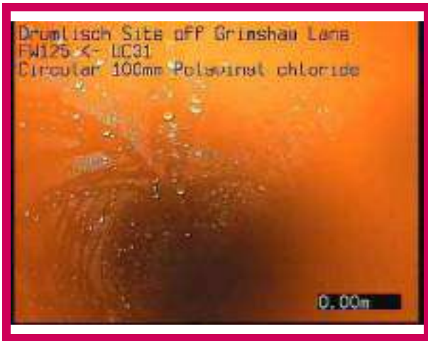
1, 00:00:00, 0.00 m Start node, manhole, reference: FW125
