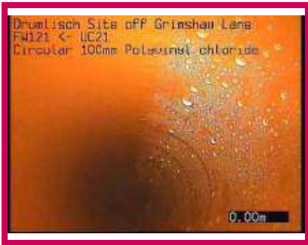
1, 00:00:00, 0.00 m Start node, manhole, reference: FW121
