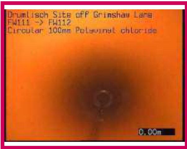
1, 00:00:00, 0.00 m Start node, manhole, reference: FW111
