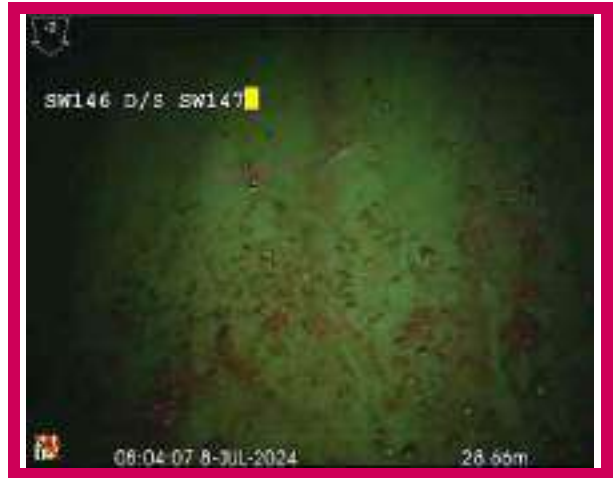
2, 00:01:23, 28.62 m Finish node, manhole, reference: SW147
