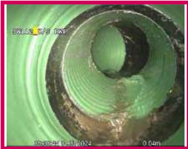
1, 00:00:00, 0.00 m Start node, manhole, reference: SW112
