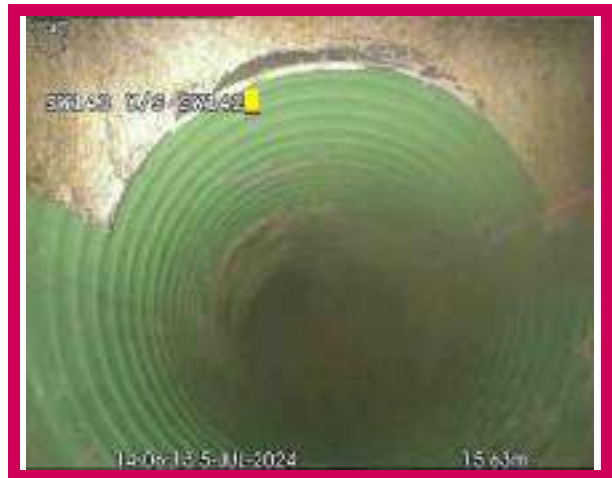
2, 00:00:59, 15.63 m Finish node, manhole, reference: SW142
