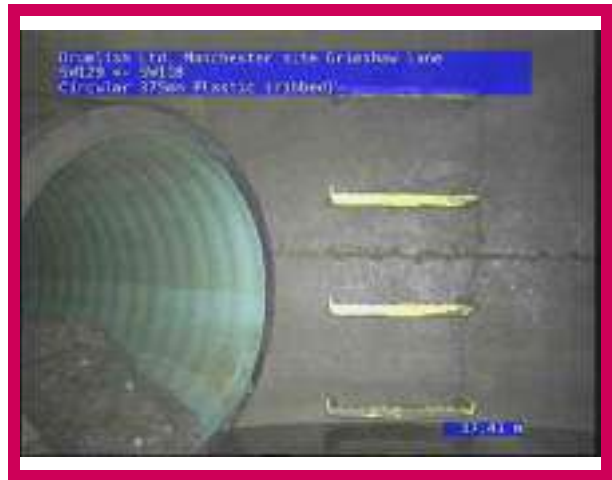
2, 00:02:29, 37.41 m Finish node, catchpit, reference: SW129
