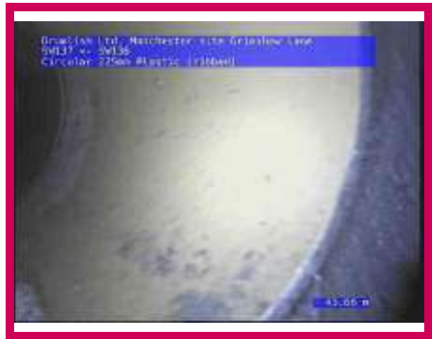
2, 00:02:31, 43.66 m Finish node, manhole, reference: SW136
