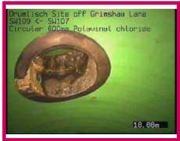
2, 00:01:29, 18.88 m Connection other than junction at 11 o'clock, 150mm dia
