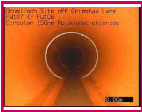
1, 00:00:00, 0.00 m Start node, manhole, reference: FW107
