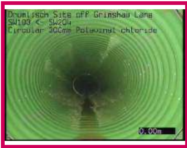
1, 00:00:00, 0.00 m Start node, manhole, reference: SW103
