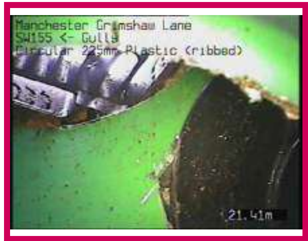
2, 00:03:39, 21.41 m Finish node, other special chamber, reference: Gully, In gully
