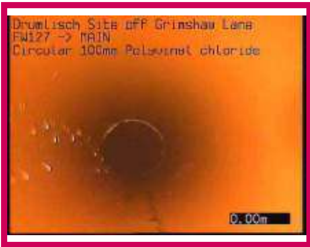
1, 00:00:00, 0.00 m Start node, manhole, reference: FW127
