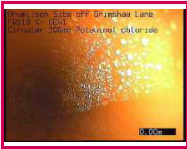
1, 00:00:00, 0.00 m Start node, manhole, reference: FW119
