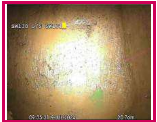
2, 00:01:01, 20.76 m Finish node, manhole, reference: SW131
