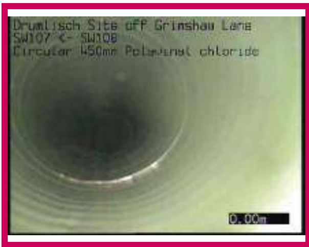
1, 00:00:00, 0.00 m Start node, manhole, reference: SW107
