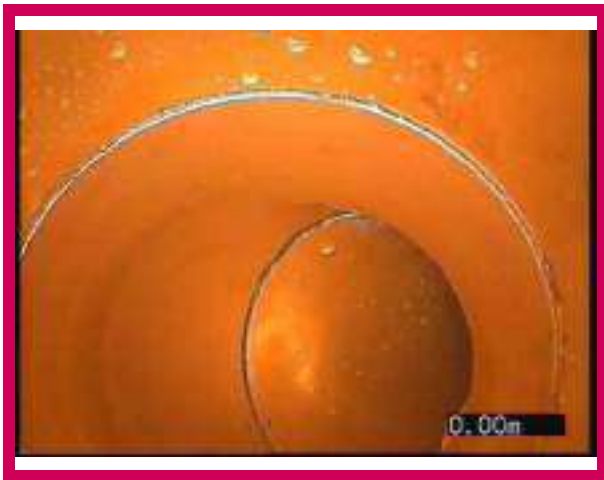
1, 00:00:00, 0.00 m Start node, manhole, reference: FW102
