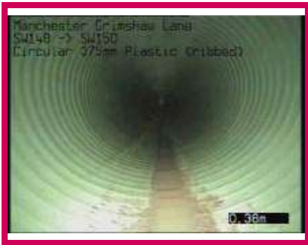
1, 00:00:00, 0.00 m Start node, manhole, reference: SW148
