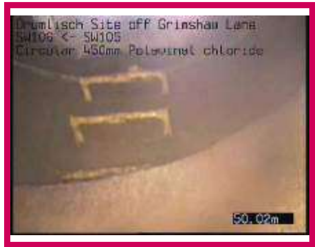
2, 00:03:17, 50.02 m Finish node, manhole, reference: SW105
