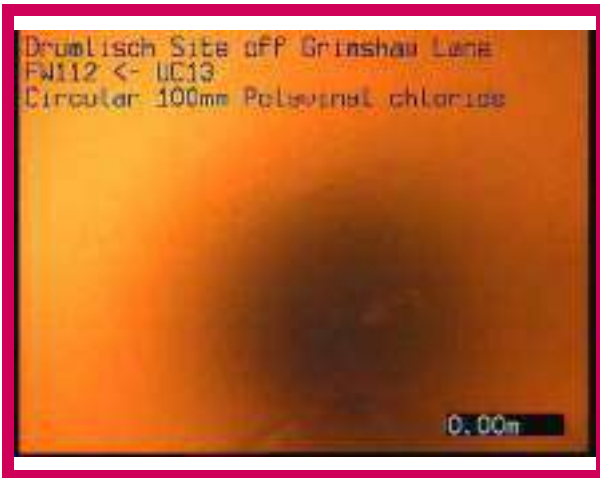
1, 00:00:00, 0.00 m Start node, manhole, reference: FW112
