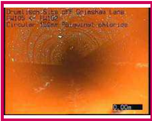
1, 00:00:00, 0.00 m Start node, manhole, reference: FW105
