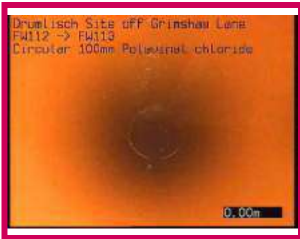
1, 00:00:00, 0.00 m Start node, manhole, reference: FW112
