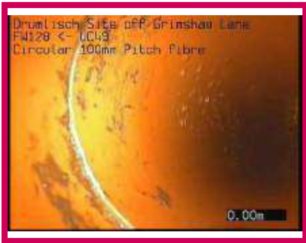
1, 00:00:00, 0.00 m Start node, manhole, reference: FW128
