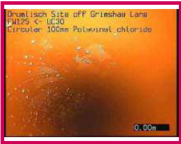
1, 00:00:00, 0.00 m Start node, manhole, reference: FW125
