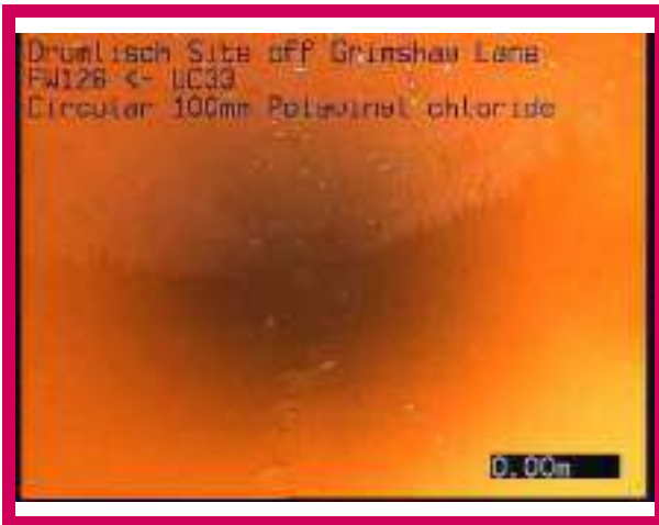
1, 00:00:00, 0.00 m Start node, manhole, reference: FW126
