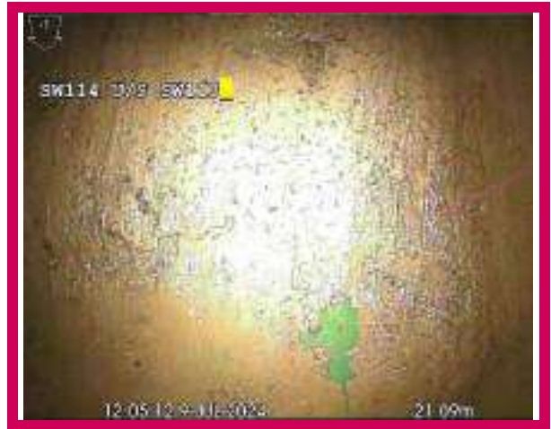
2, 00:01:35, 21.09 m Finish node, manhole, reference: SW113
