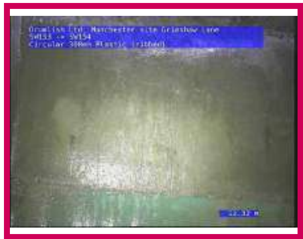
2, 00:00:40, 12.32 m Finish node, manhole, reference: SW154
