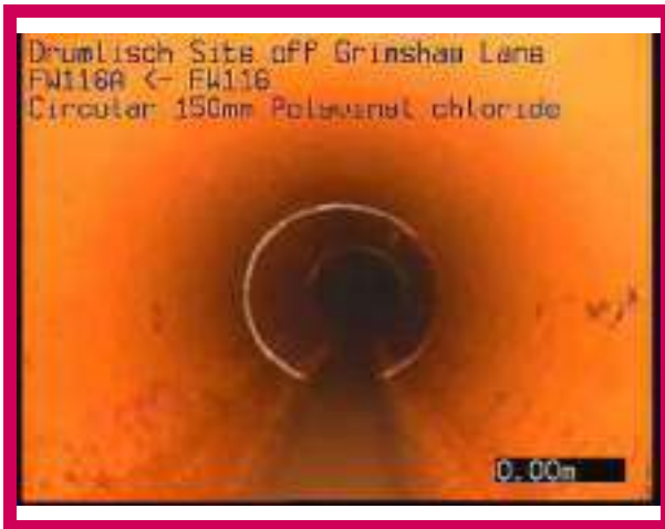
1, 00:00:00, 0.00 m Start node, manhole, reference: FW116A
