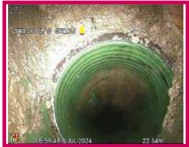
2, 00:01:03, 22.54 m Finish node, manhole, reference: SW135
