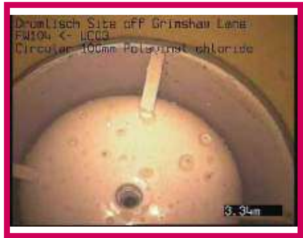
2, 00:00:23, 3.34 m Finish node, other special chamber, reference: UC03, HOS
