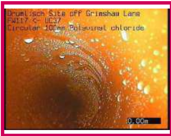
1, 00:00:00, 0.00 m Start node, manhole, reference: FW117
