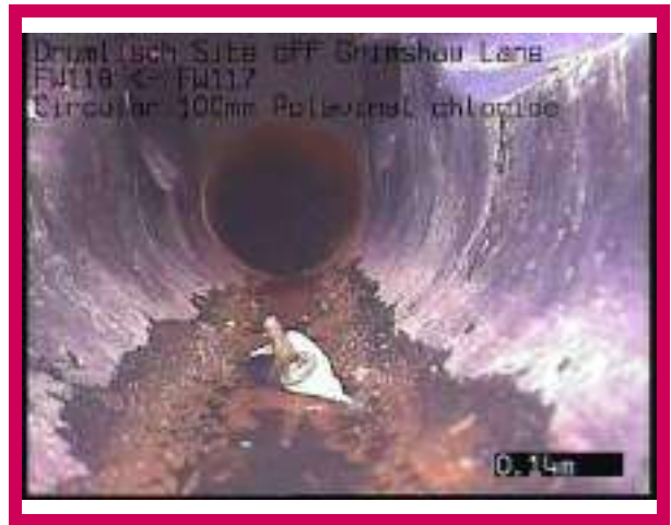
2, 00:00:17, 0.14 m Finish node, manhole, reference: FW117
