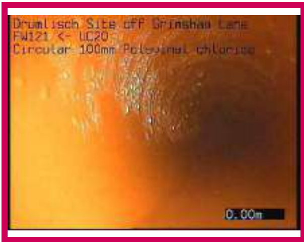
1, 00:00:00, 0.00 m Start node, manhole, reference: FW121
