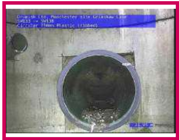
2, 00:01:49, 21.96 m Finish node, catchpit, reference: SW138
