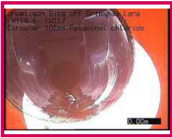
1, 00:00:00, 0.00 m Start node, manhole, reference: FW118
