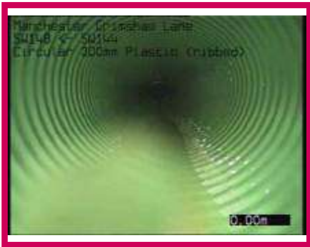
1, 00:00:00, 0.00 m Start node, manhole, reference: SW148
