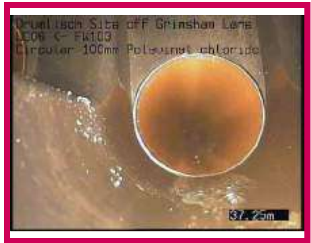
2, 00:02:36, 37.25 m Finish node, manhole, reference: FW103
