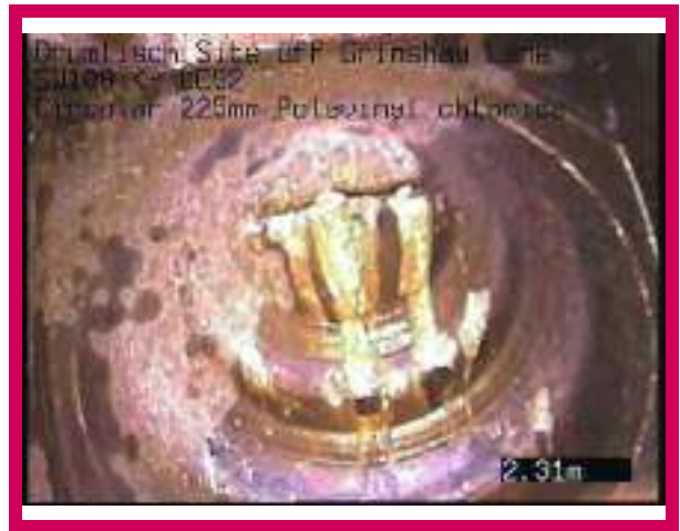
2, 00:00:31, 2.31 m Finish node, gully, reference: UC52, Gully
