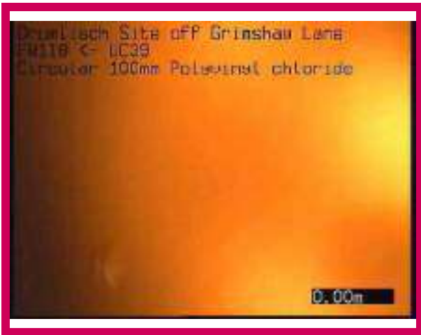
1, 00:00:00, 0.00 m Start node, manhole, reference: FW118
