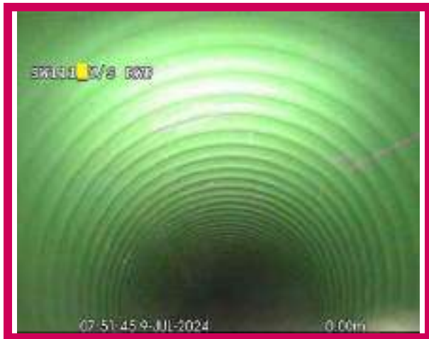
1, 00:00:00, 0.00 m Start node, manhole, reference: SW111
