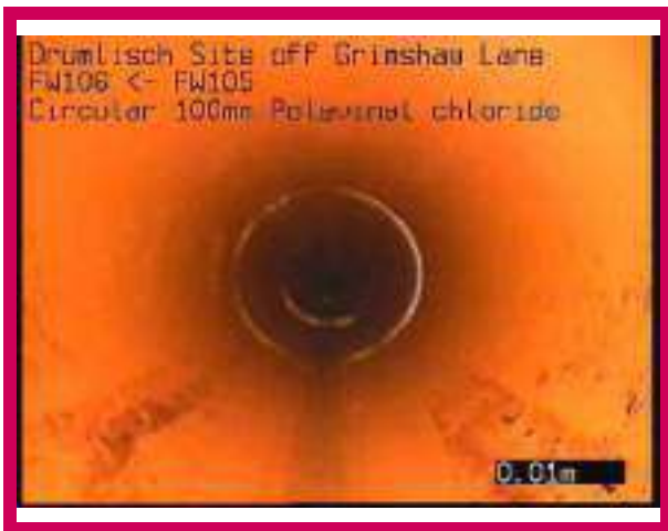
1, 00:00:00, 0.00 m Start node, manhole, reference: FW106
