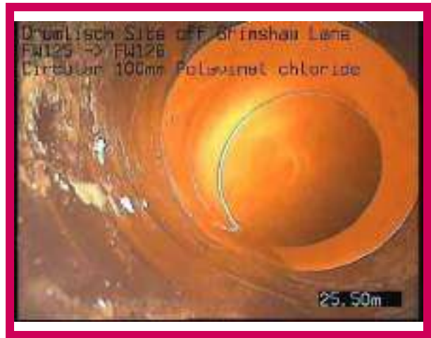
2, 00:01:47, 25.50 m Finish node, manhole, reference: FW126
