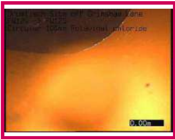
1, 00:00:00, 0.00 m Start node, manhole, reference: FW124
