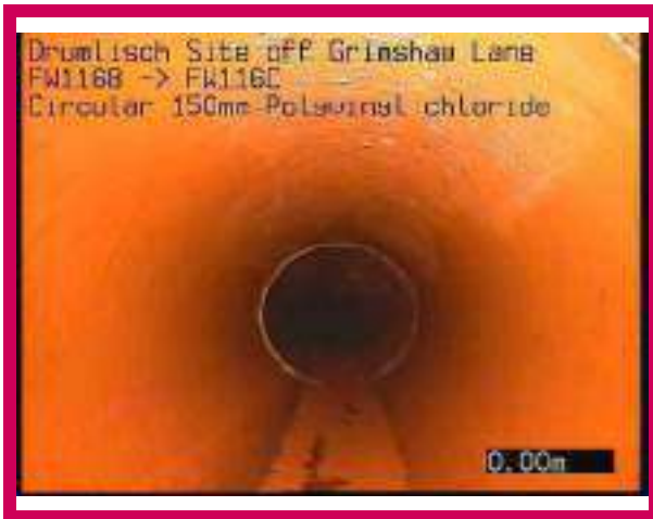
1, 00:00:00, 0.00 m Start node, manhole, reference: FW116B
