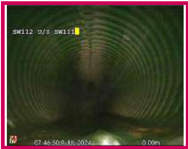
1, 00:00:00, 0.00 m Start node, manhole, reference: SW112
