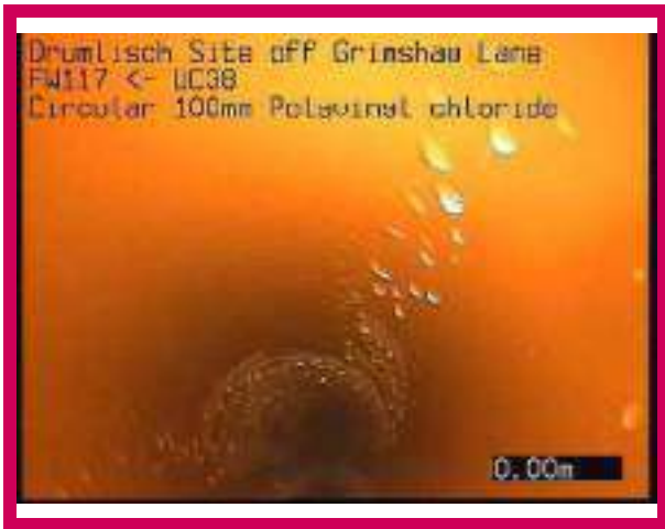
1, 00:00:00, 0.00 m Start node, manhole, reference: FW117
