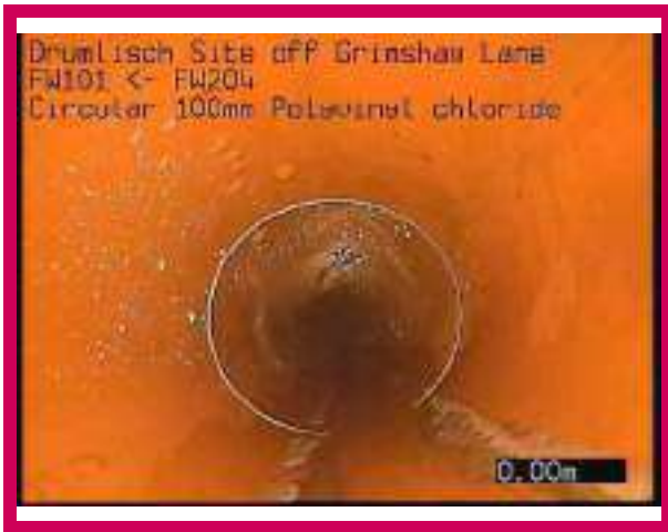
1, 00:00:00, 0.00 m Start node, manhole, reference: FW101
