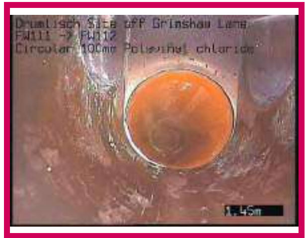
2, 00:00:14, 1.45 m Finish node, manhole, reference: FW112, FW112
