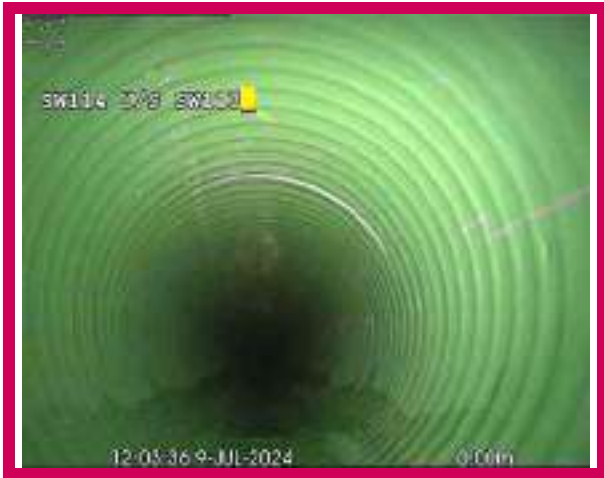
1, 00:00:00, 0.00 m Start node, manhole, reference: SW114
