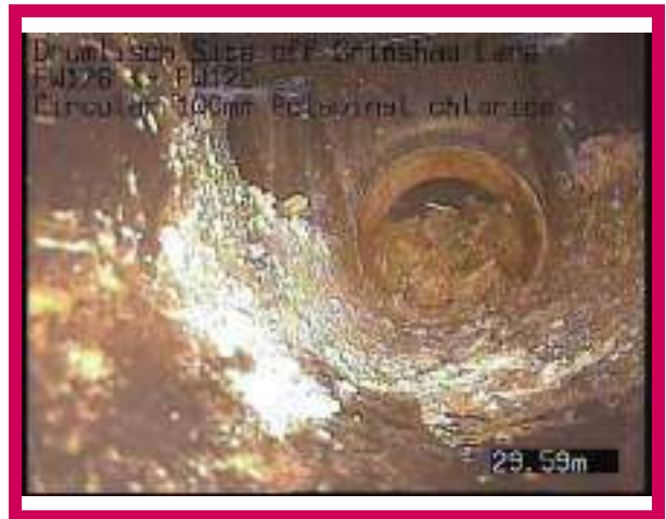
2, 00:02:02, 29.59 m Finish node, manhole, reference: FW120
