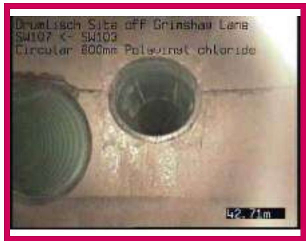
2, 00:02:39, 42.71 m Finish node, catchpit, reference: SW103
