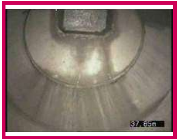
2, 00:03:03, 37.93 m Finish node, manhole, reference: SW126
