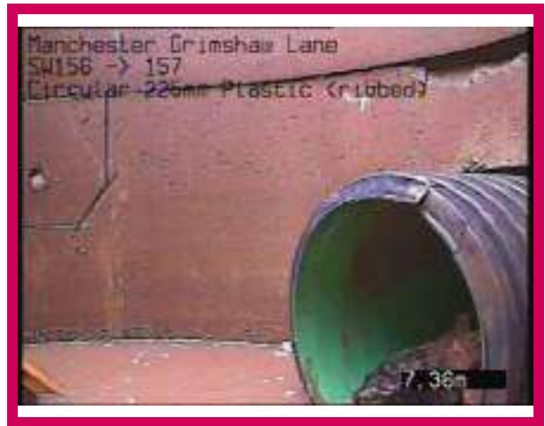
2, 00:00:53, 7.36 m Finish node, manhole, reference: SW157
