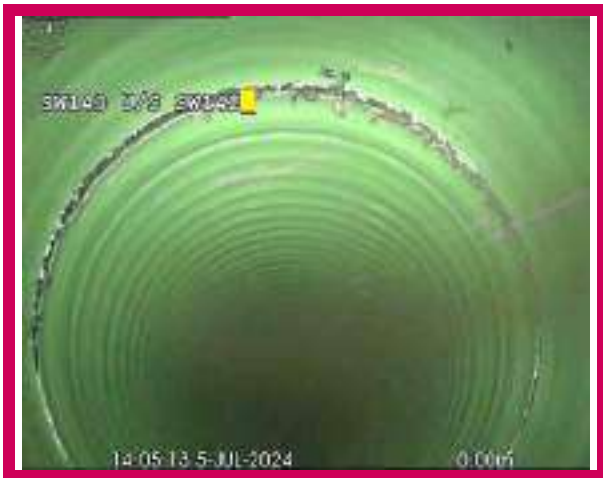
1, 00:00:00, 0.00 m Start node, manhole, reference: SW143
