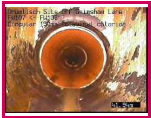
2, 00:04:09, 41.94 m Finish node, manhole, reference: FW106
