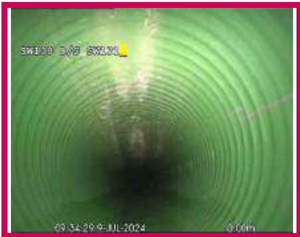
1, 00:00:00, 0.00 m Start node, manhole, reference: SW130
