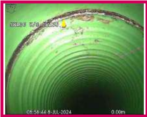
1, 00:00:00, 0.00 m Start node, manhole, reference: SW136
