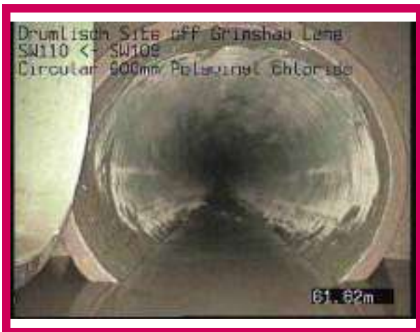
3, 00:04:32, 61.82 m Finish node, catchpit, reference: SW109
