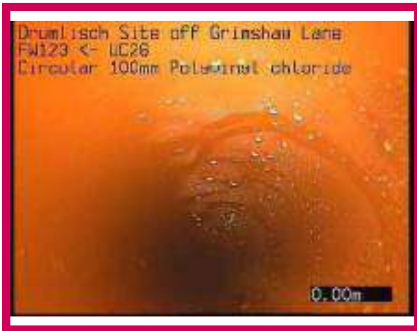
1, 00:00:00, 0.00 m Start node, manhole, reference: FW123
