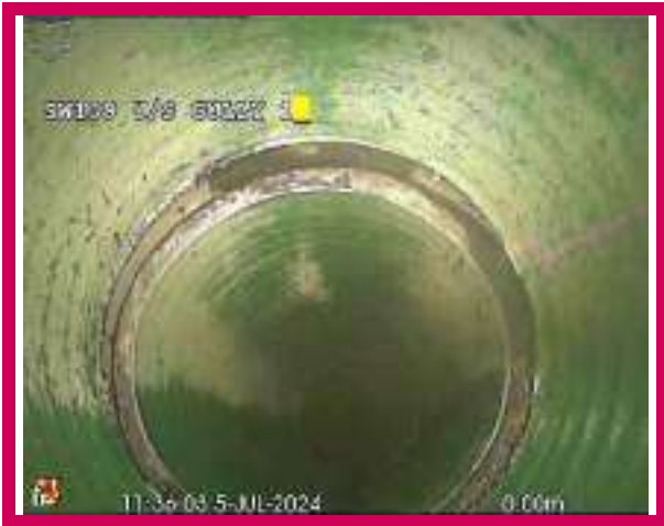
1, 00:00:00, 0.00 m Start node, manhole, reference: SW139
