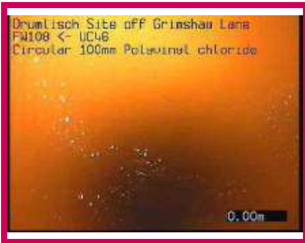
1, 00:00:00, 0.00 m Start node, manhole, reference: FW108
