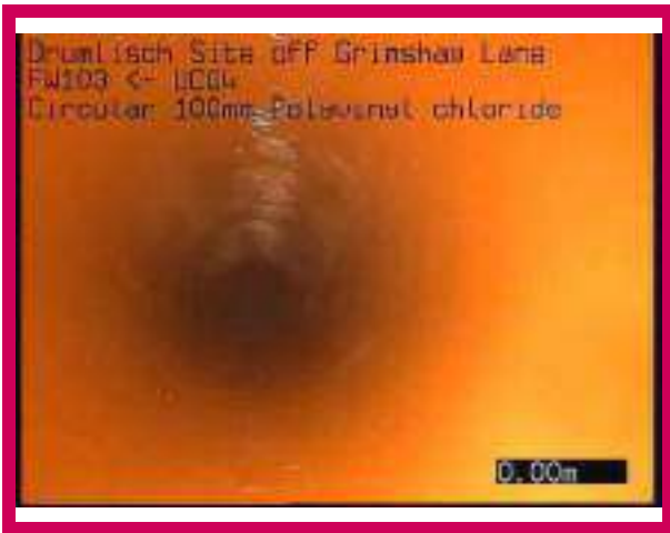
1, 00:00:00, 0.00 m Start node, manhole, reference: FW103
