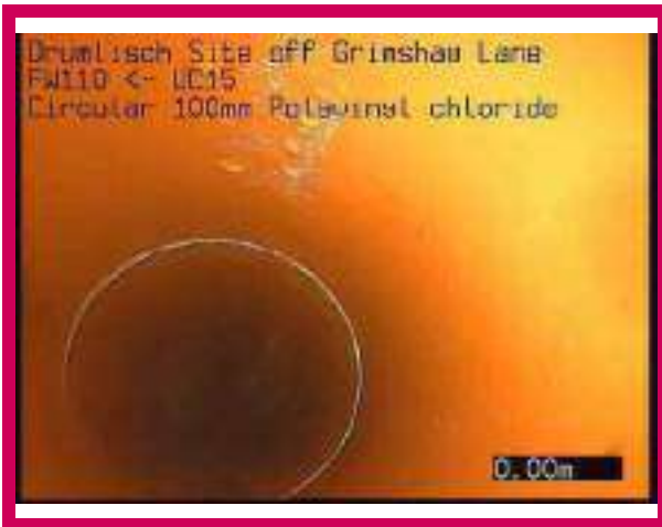
1, 00:00:00, 0.00 m Start node, manhole, reference: FW110
