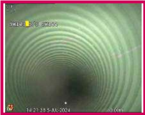
1, 00:00:00, 0.00 m Start node, manhole, reference: SW143
