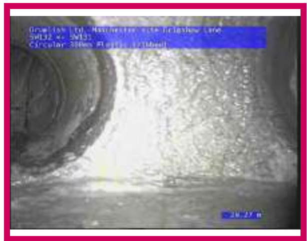
2, 00:02:02, 29.27 m Finish node, manhole, reference: SW131
