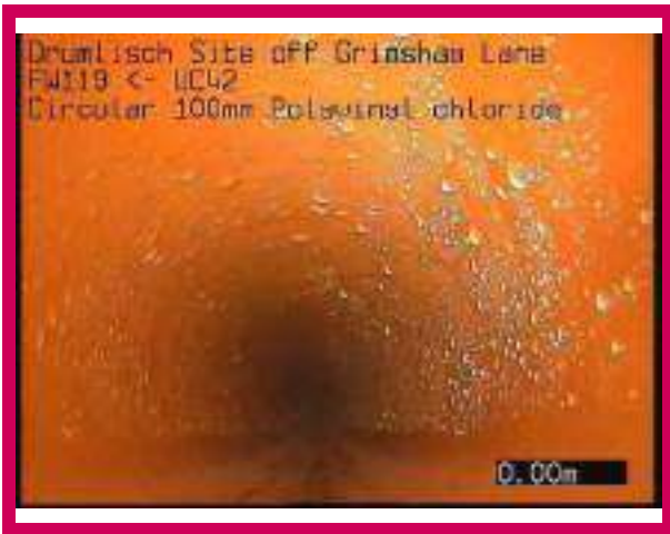
1, 00:00:00, 0.00 m Start node, manhole, reference: FW119
