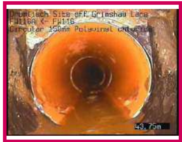
2, 00:04:40, 43.75 m Finish node, manhole, reference: FW116
