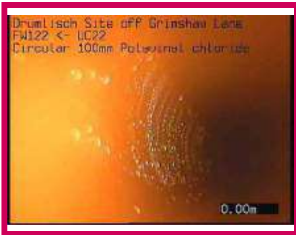
1, 00:00:00, 0.00 m Start node, manhole, reference: FW122
