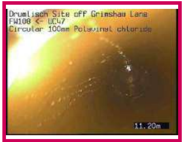
2, 00:01:08, 11.20 m Finish node, other special chamber, reference: UC47, In View
