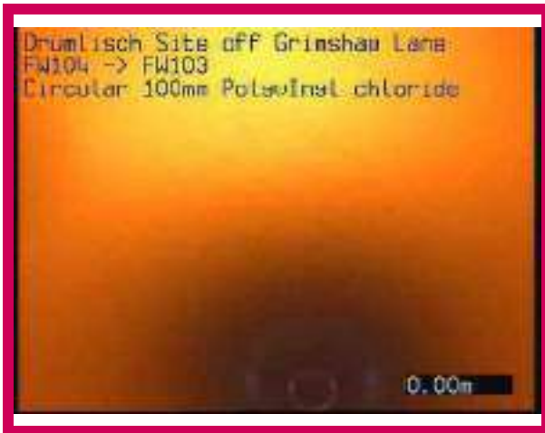
1, 00:00:00, 0.00 m Start node, manhole, reference: FW104
