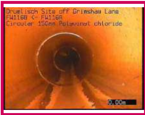
1, 00:00:00, 0.00 m Start node, manhole, reference: FW116B
