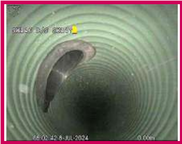
1, 00:00:00, 0.00 m Start node, manhole, reference: SW147
