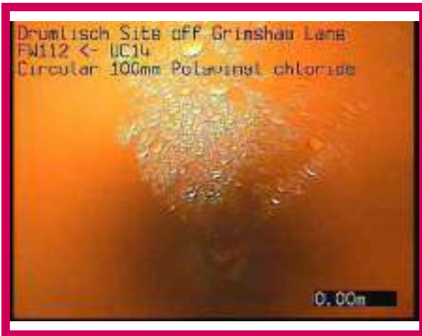
1, 00:00:00, 0.00 m Start node, manhole, reference: FW112
