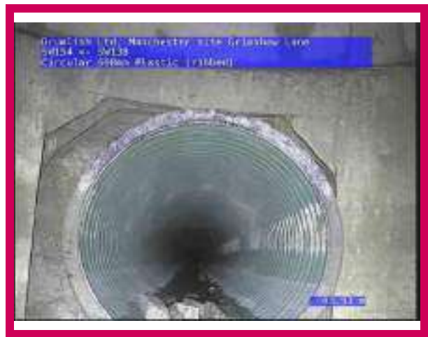
2, 00:03:10, 43.51 m Finish node, catchpit, reference: SW138
