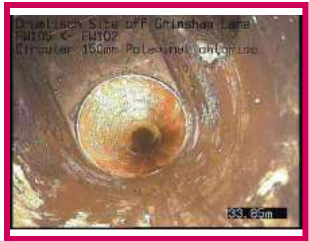
2, 00:03:03, 33.85 m Finish node, manhole, reference: FW102
