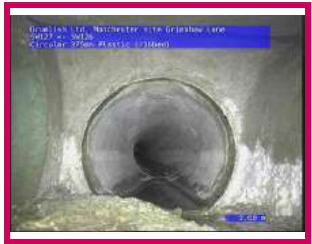
2, 00:00:15, 3.68 m Finish node, manhole, reference: SW126
