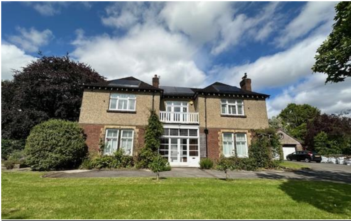
Fig.1 The principal elevation of Stenner Brow
