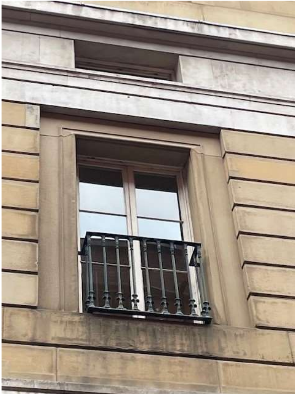
Essex Street Balcony Doors (External)
