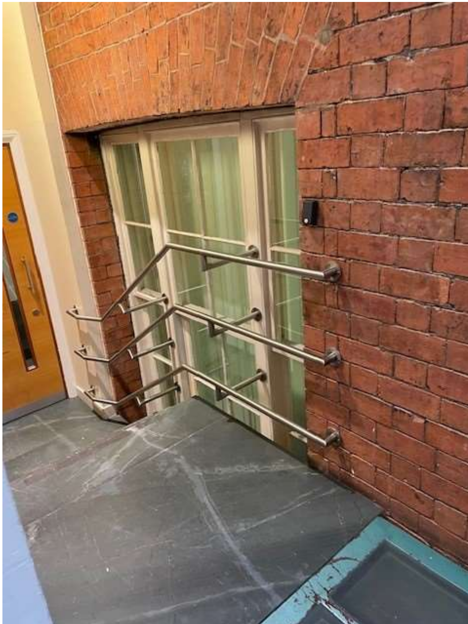
Window 1 (External Before 1995 Refurbishment).
