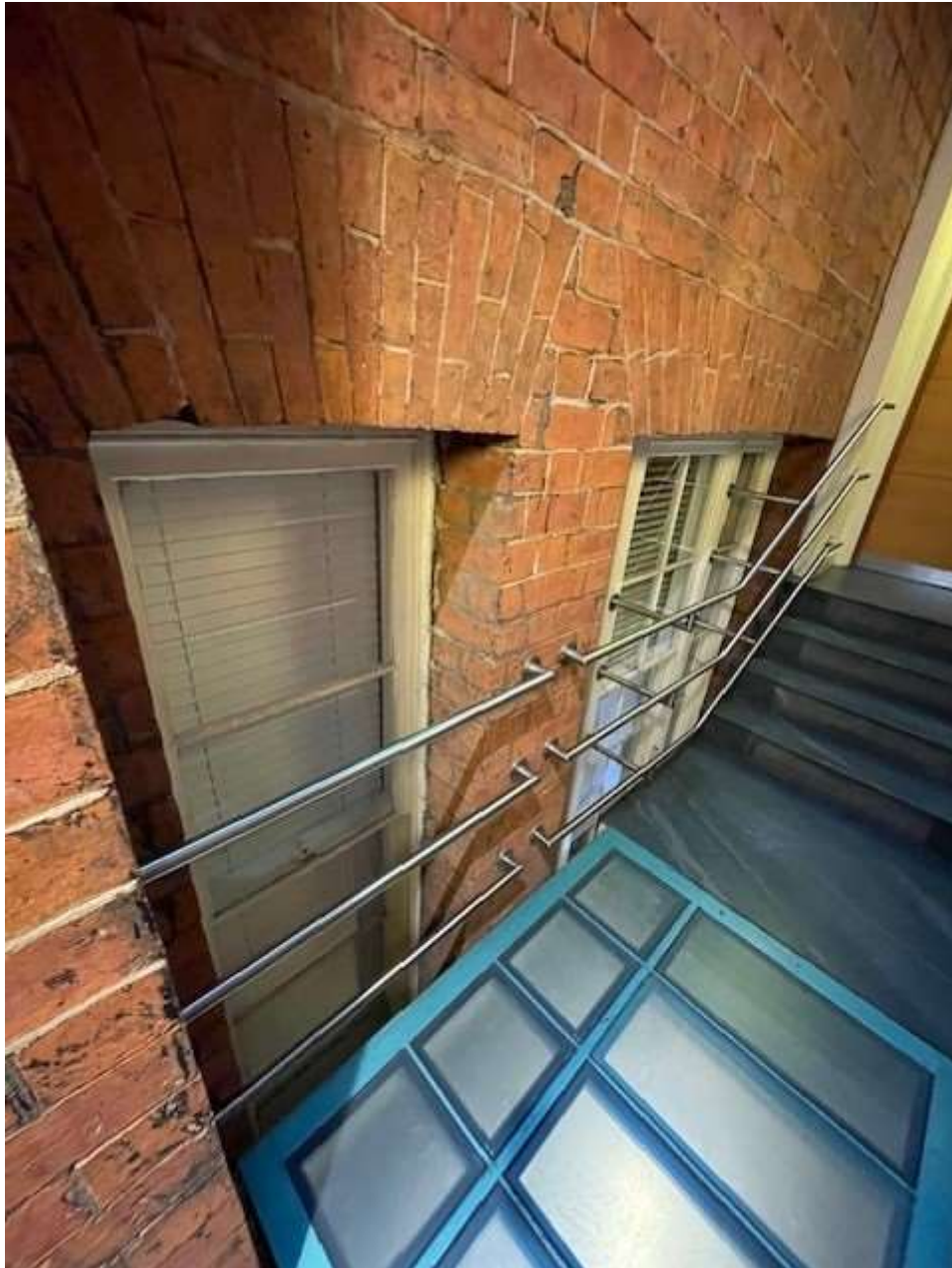
No. 2 Windows (External Before 1995 Refurbishment).
