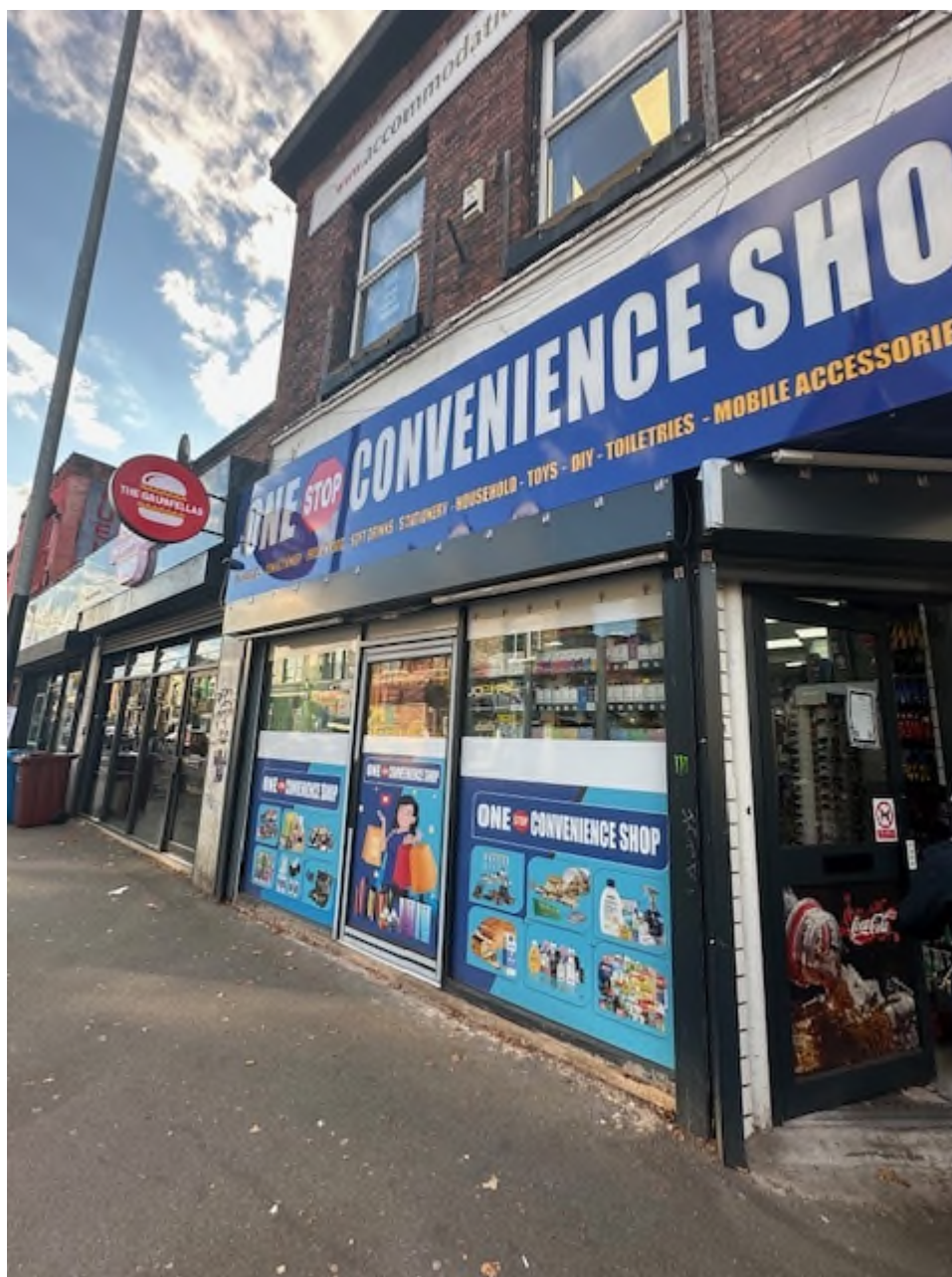
Figure 2. The application property principal elevation, October 2024
