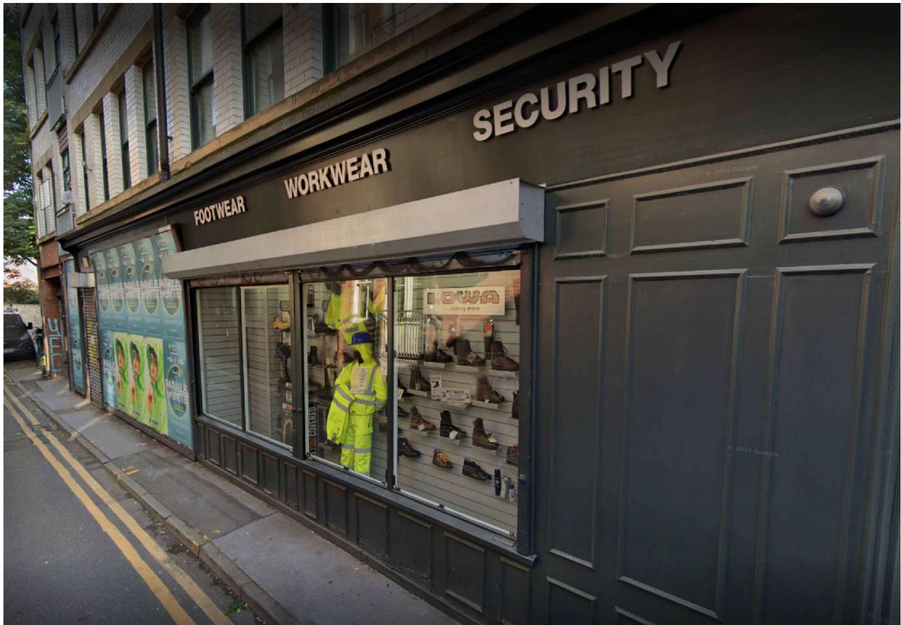
PHOTOS AS EXISTING ELEVATION A
