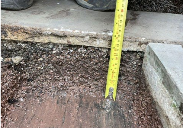
Figure 3: Image of paving build up and levels survey
