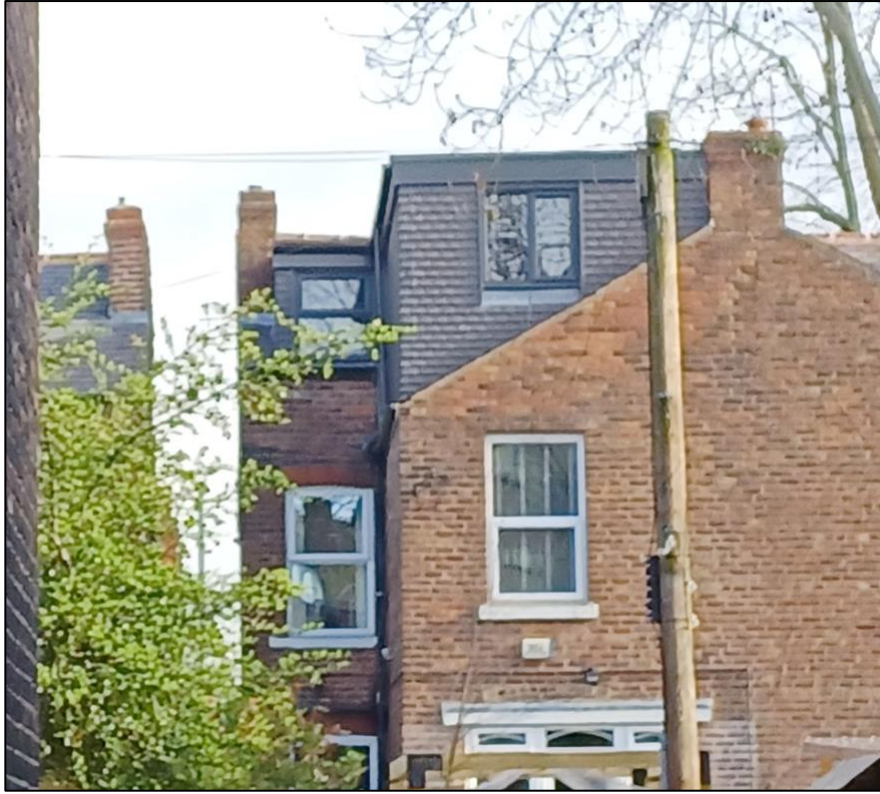
Figure 3: Image of the roof extension to which this appeal relates.
