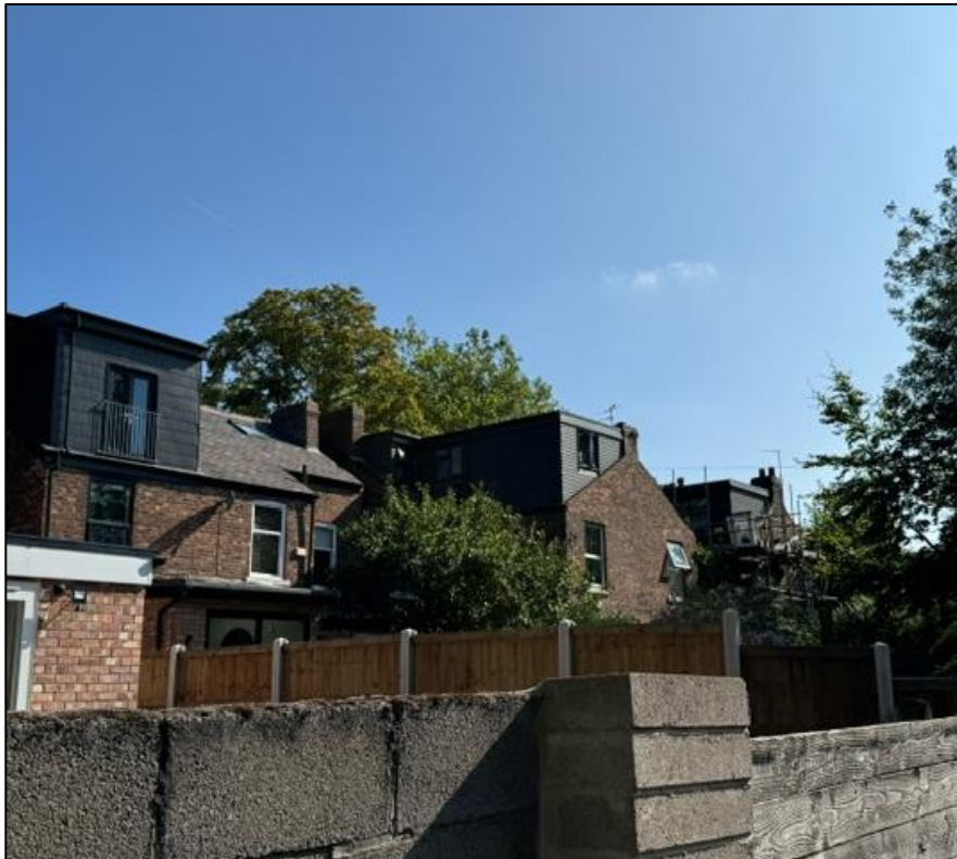
Figure 5: Photograph of dormers at numbers 19, 23 and 27.
