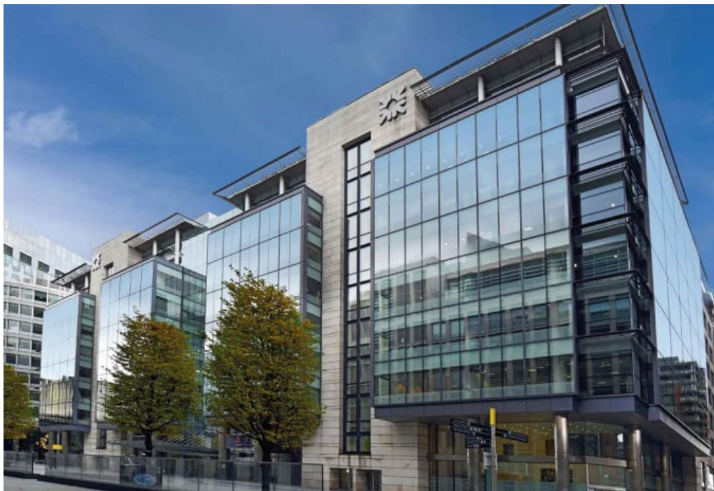
Figure 2.1: 1 Hardman Boulevard, existing view from Left Bank
