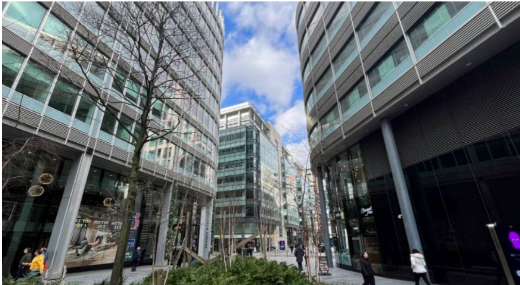
Figure 2.2: 1 Hardman Boulevard, existing view from Hardman Square
