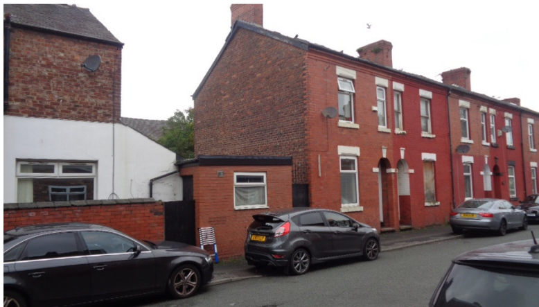
Adjoining Elevation of Application Property.
