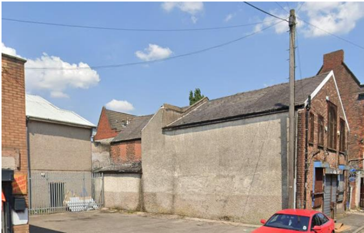
View of the side of the building from Lockett Street
