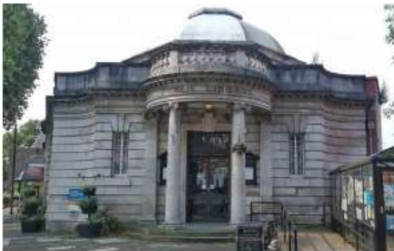
The entrance portico, north elevation.
