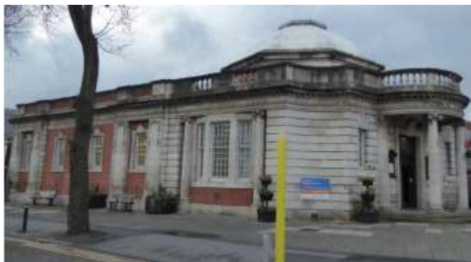
Portland stone and small gauge brickwork, east elevation.
