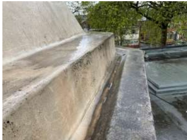
Asphalt covering to dome and perimeter gutter, note outlet in corner to gargoyle which spills over the lower roof, and infilled lantern on roof beyond.
