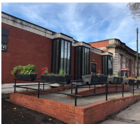
The east elevation of the 1964 extension to the library building.
