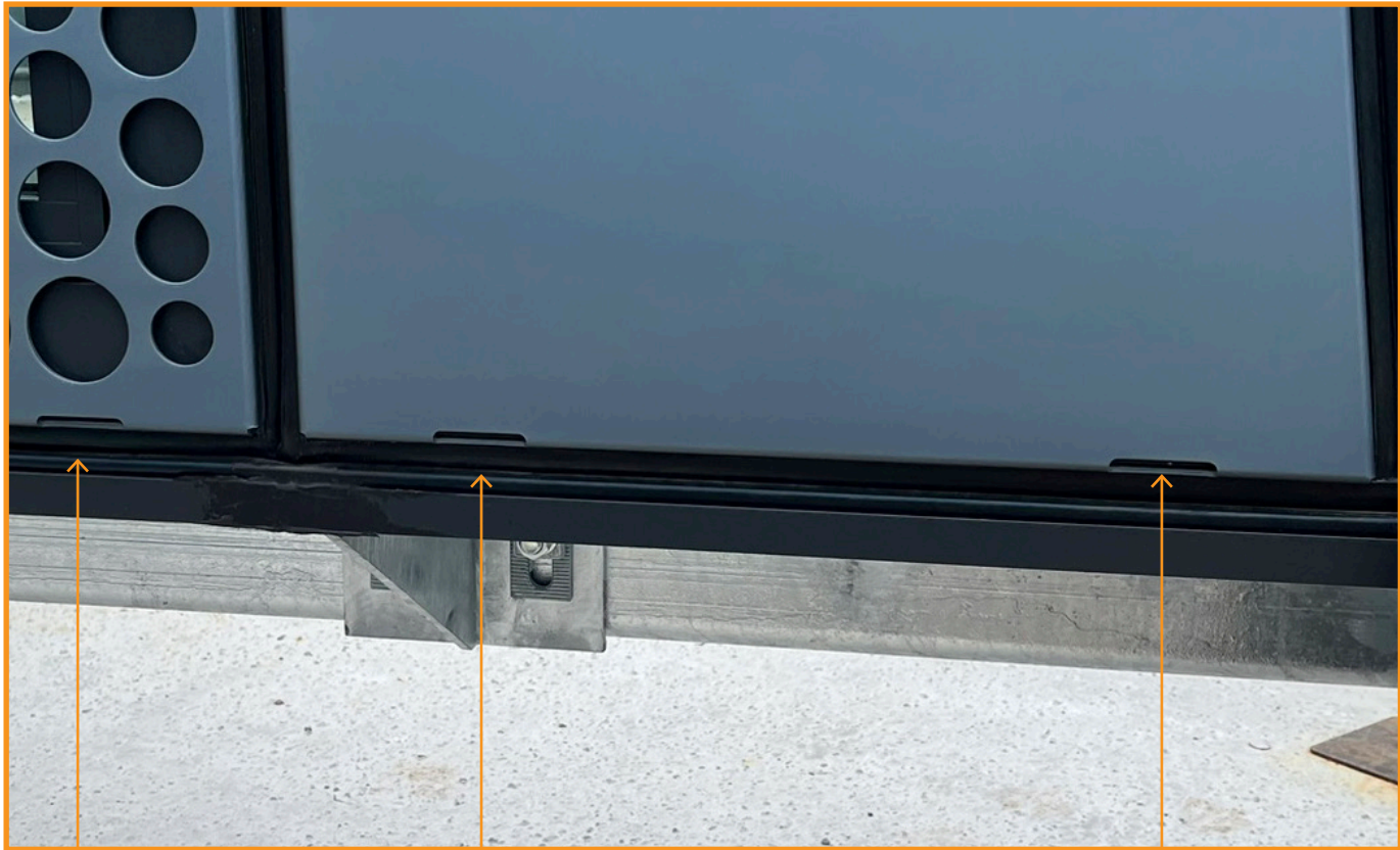
Drainage slot Drainage slot Drainage slot
