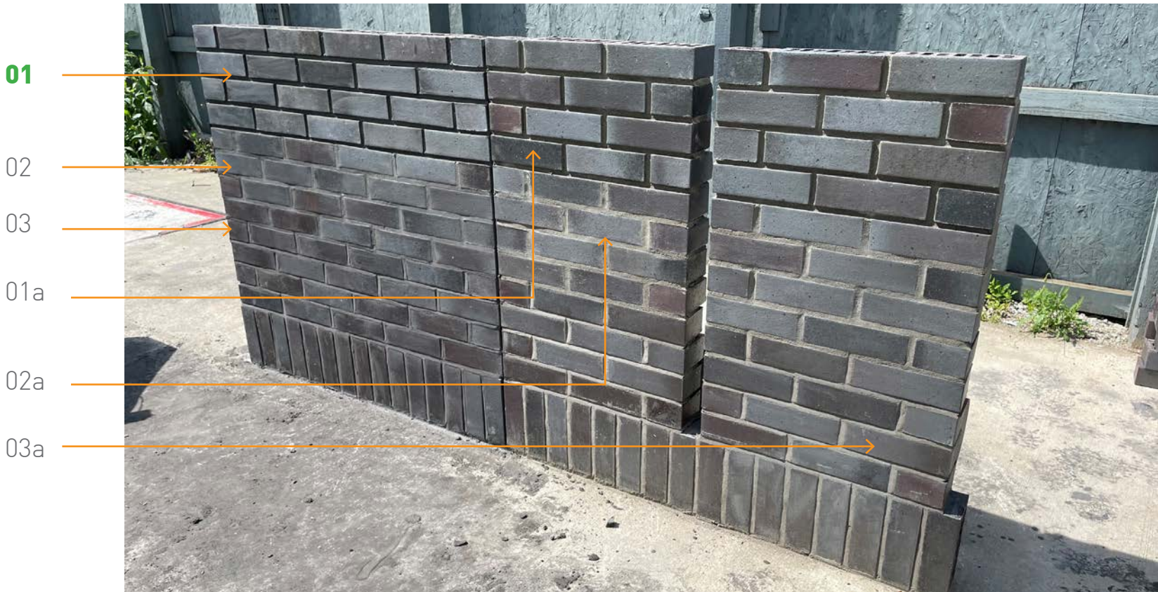
Final sample panel illustrating chosen, brick, pointing type and mortar.
