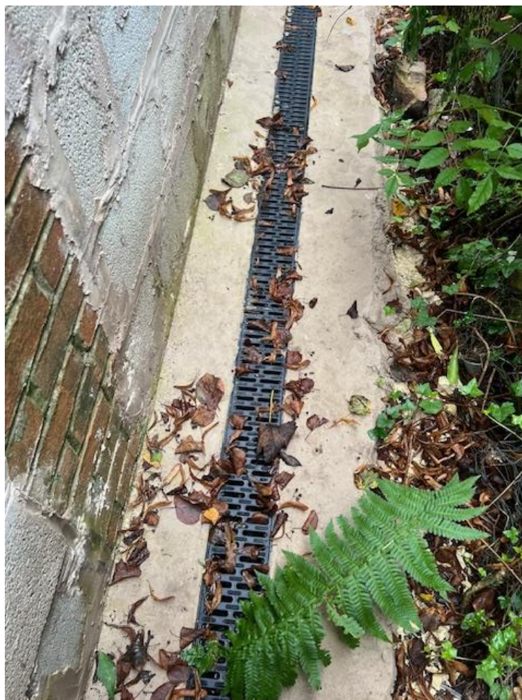
Drainage channels installed
