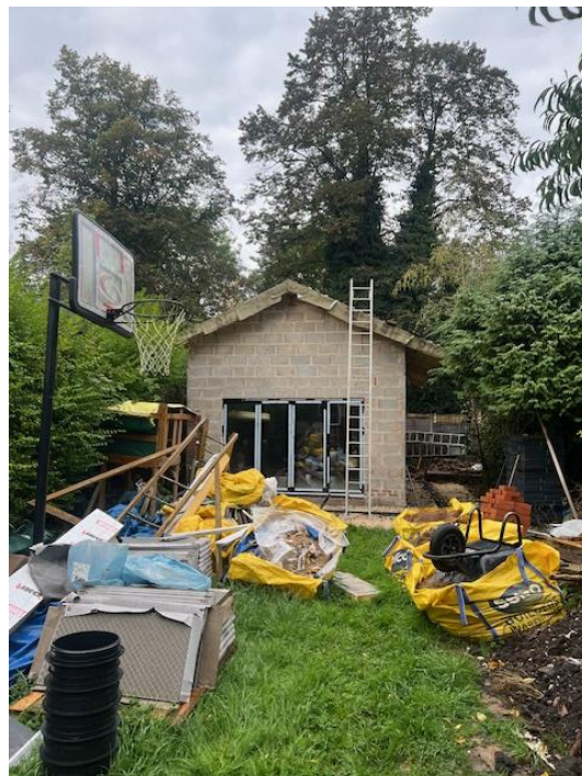
Partially constructed outbuilding
