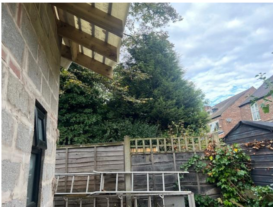
Existing boundary fence between the appeal site and southern most part of the rear garden to No. 34 Mauldeth Road. Outbuilding visible to the left and mature trees within rear garden of No. 1 Alan Road visible in the centre
