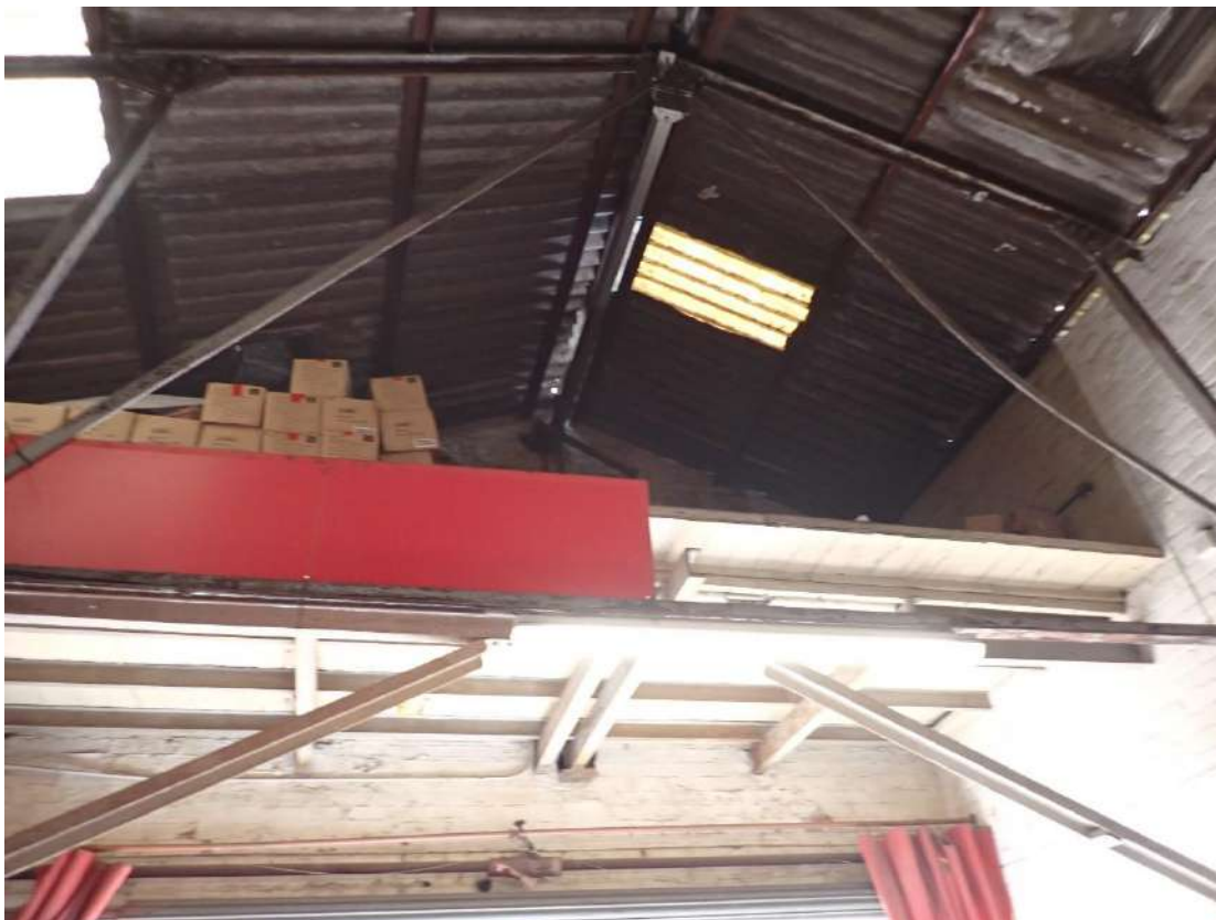
Photograph 14 – Internal view of Section 2 of the building.
