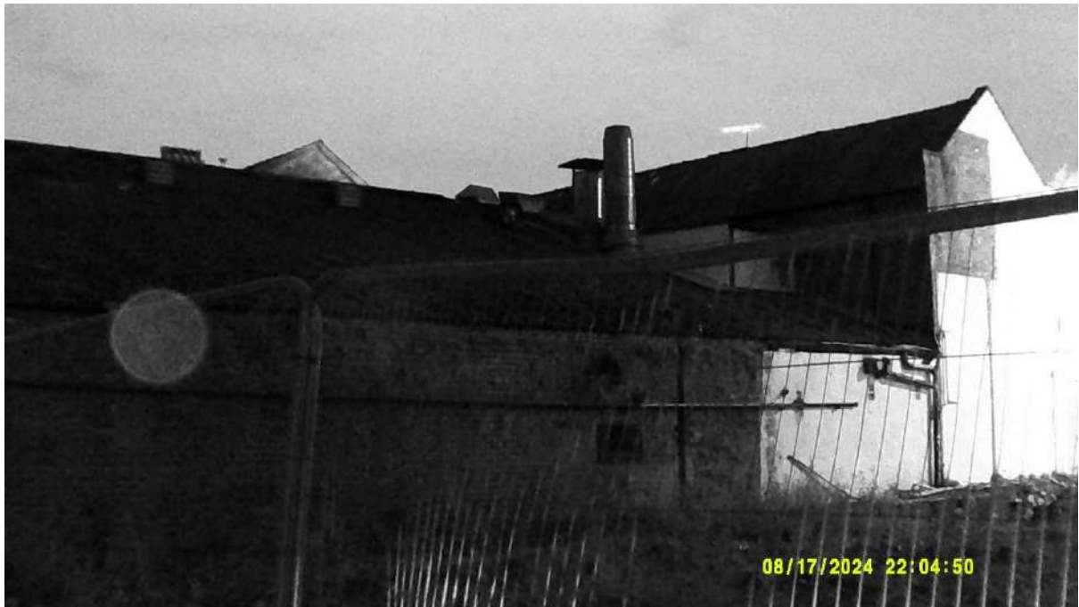
Photograph 3 – Infrared image of the southern aspect of the building taken at the darkest point of the survey at 22:04 on the 17 th August 2024.
