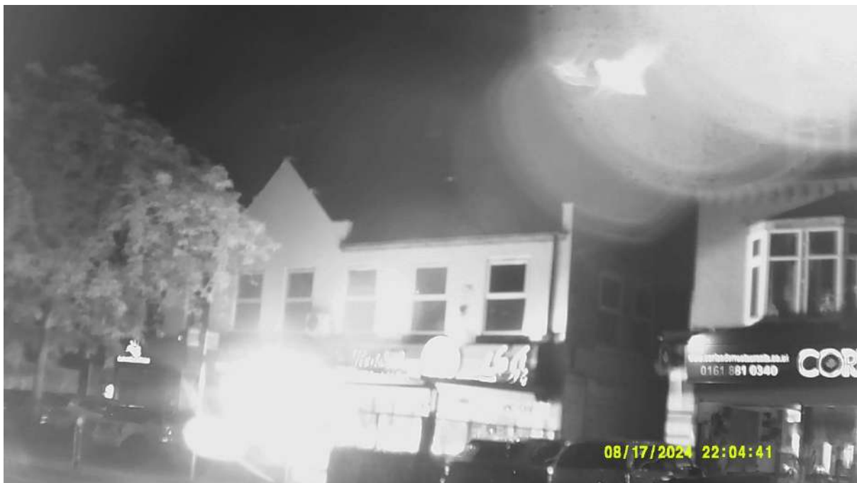
Photograph 2 – Infrared image of the eastern aspect of the building at the darkest point of the survey at 22:04 on the 17 th August 2024.
