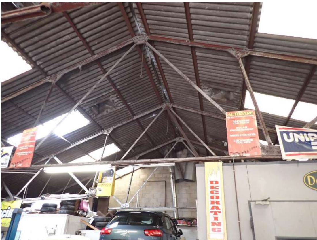
Photograph 6 – Internal view of the roof of Section 2 of the building.
