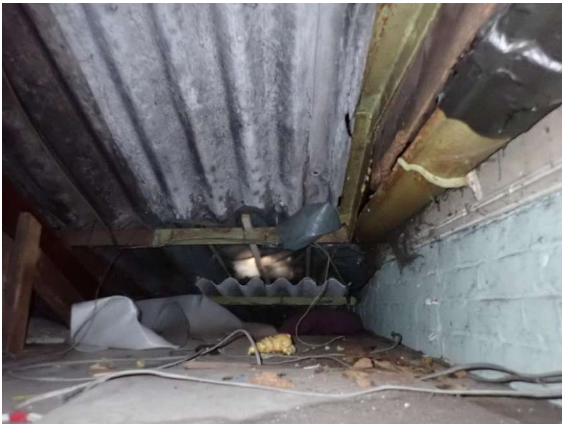
Photograph 12 – View of the light ingress in the first loft space of Section 1 of the property.
