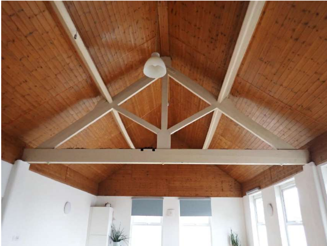
Building 9 – Interior view of the vaulted and panelled ceiling in the Yoga studio in Section 1.
