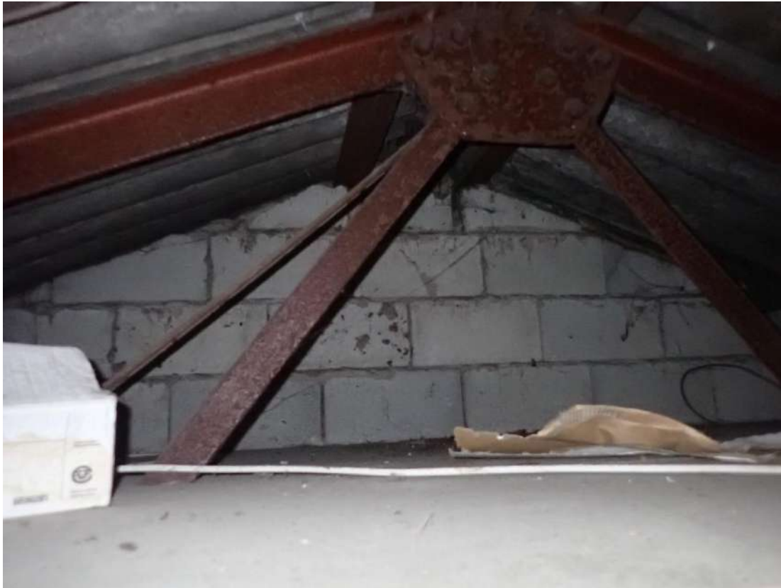
Photograph 11 – Interior view of the first loft space in section 1 of the building.
