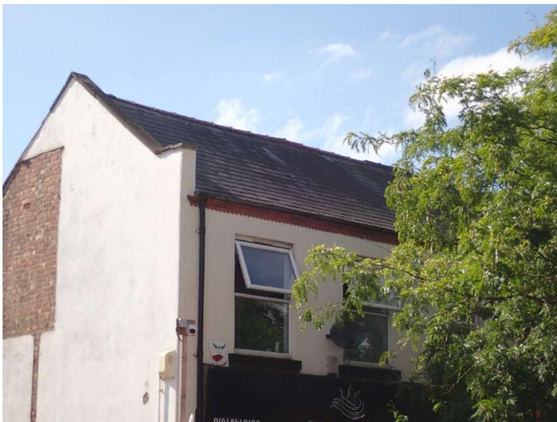
Photograph 2 – View of the southern aspect of the building showing the partial rendering.
