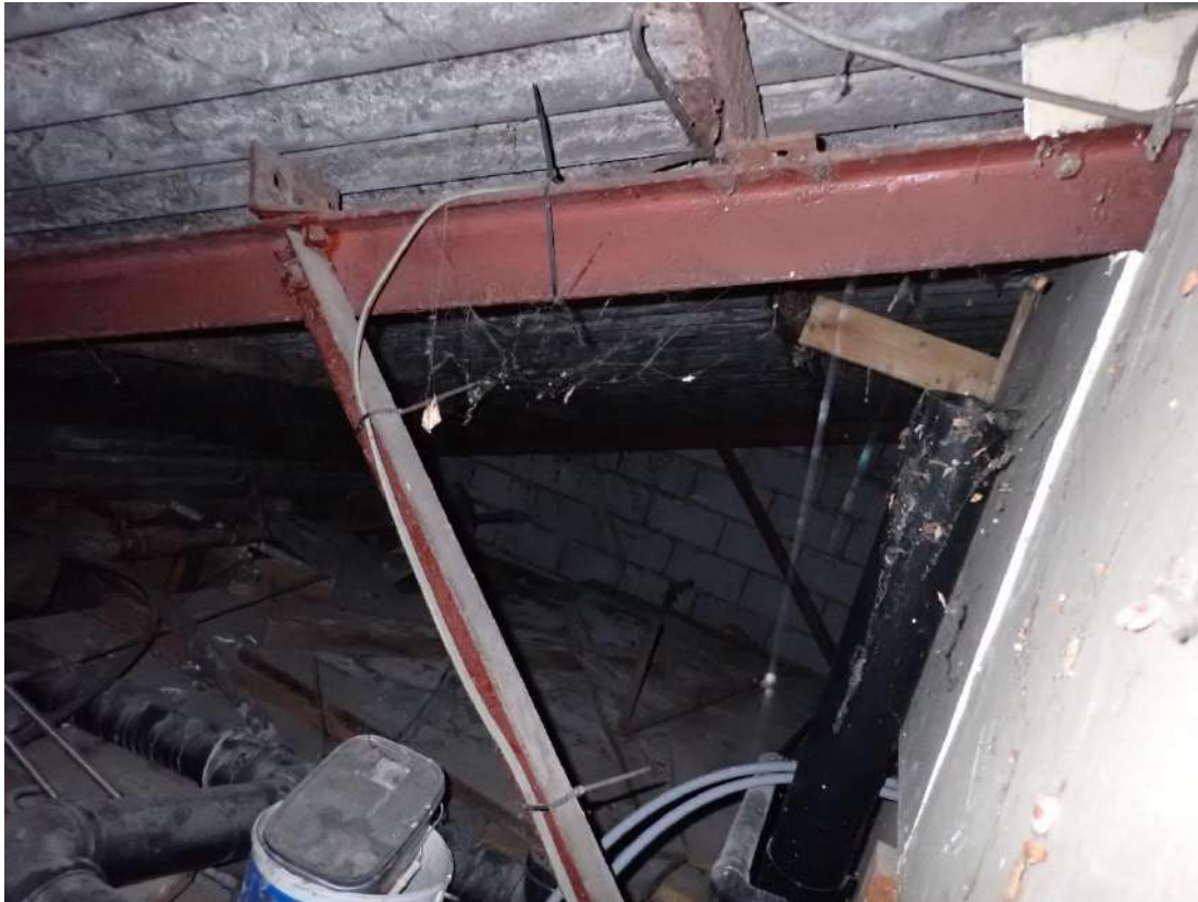
Photograph 13 – Internal view of the second loft space in Section 1.
