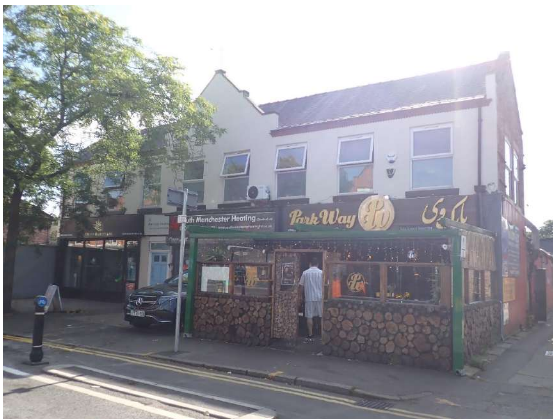
Photograph 1 – View of the eastern aspect of the building.
