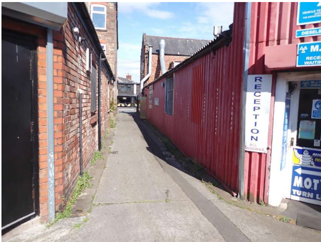
Photograph 5 – View of the metal cladding on the northern aspect of Section 2.
