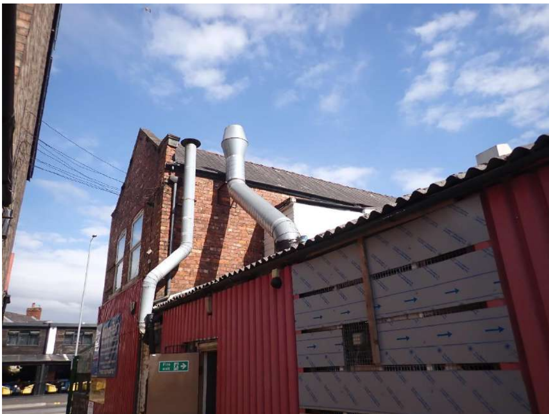
Photograph 4 – Image of the extension to the first floor on Section 1 of the building.
