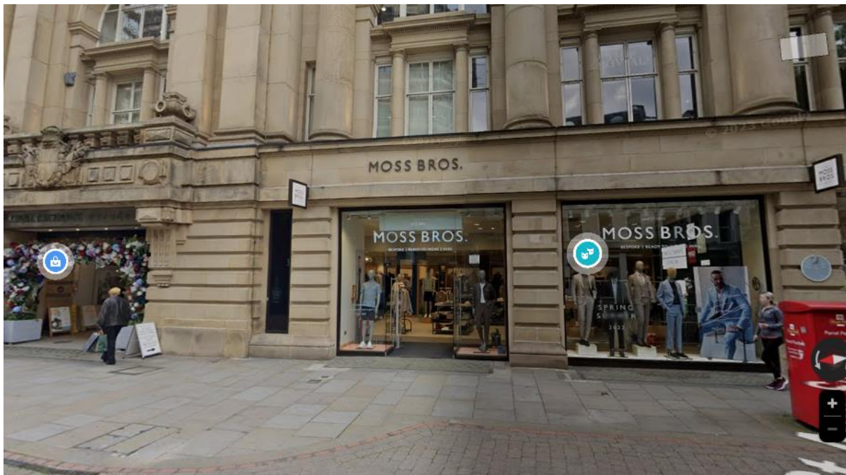
Existing Shopfront (St Ann's Square) (June 2022) (Source: Google Street View - https://maps.app.goo.gl/EWwfUMcakTnfQJoz8 )
