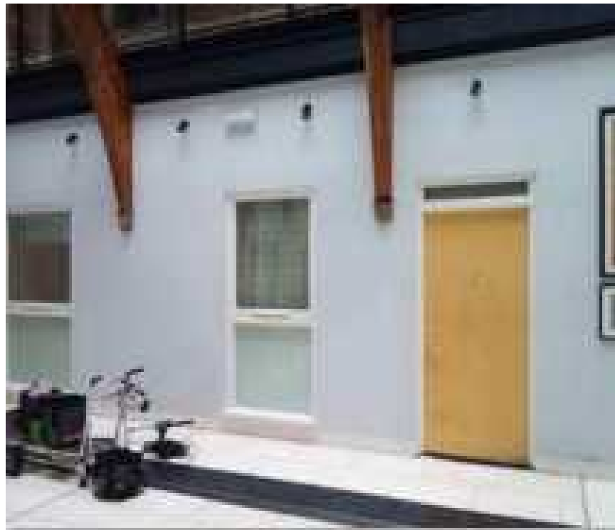
Existing Wall Type 1-Insulated Render
