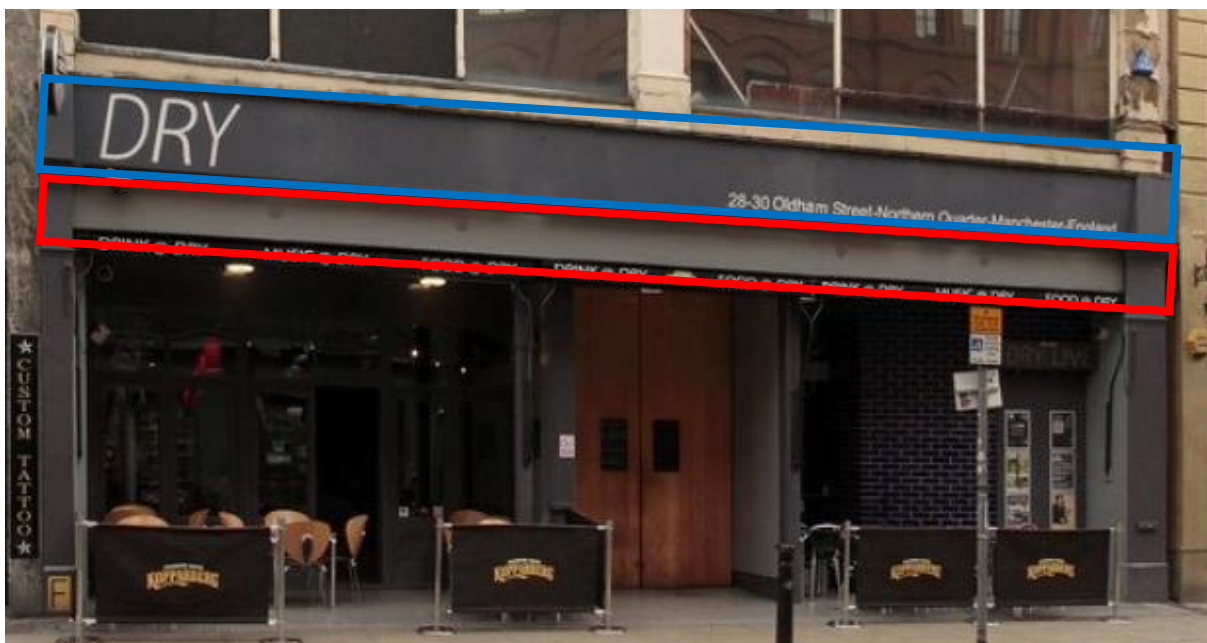
Figure 5 Existing lower and upper fascia to be cleaned, retained and decoration made good where required.
