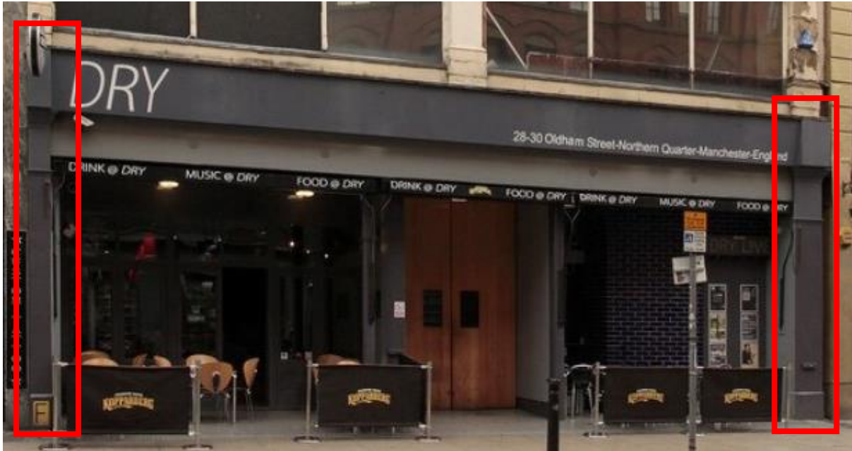
Figure 4 Existing pedestal, pilasters and bracket consoles to be cleaned and retained.
