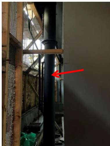
Figure 2 Existing circular columns flanking the entrance
