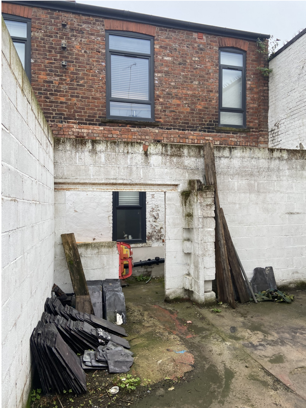
Internal walls with 12 and 12A Standish Street behind
