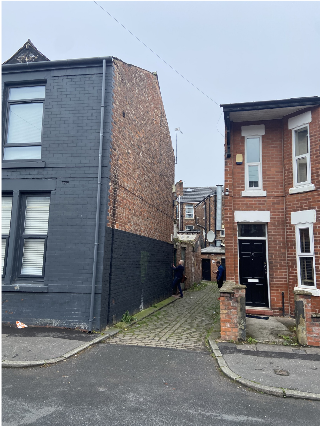
Access passageway to the site
