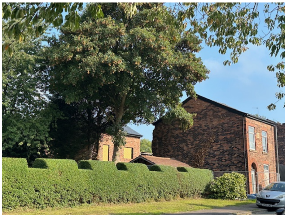
Fig.2 – Public view of application site from Holyrood Street facing north east
