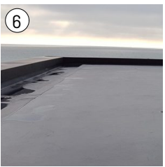
Single ply membrane roof
