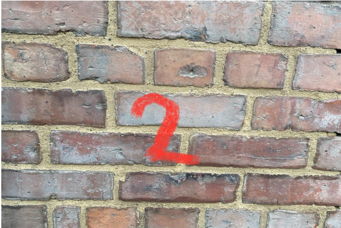
Photo 3 - Raked out cutting through the centre of the mortar with a thin blade and then taken out the mortar using handheld tools to the required depth and brushed out leaving the area clean.
