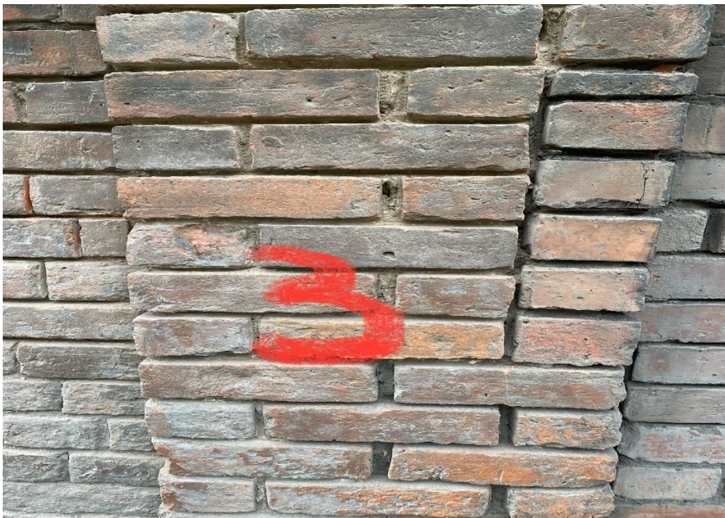
Photo 3 - Raked out cutting through the centre of the mortar with a thin blade and then taken out the mortar using handheld tools to the required depth and brushed out leaving the area clean.
