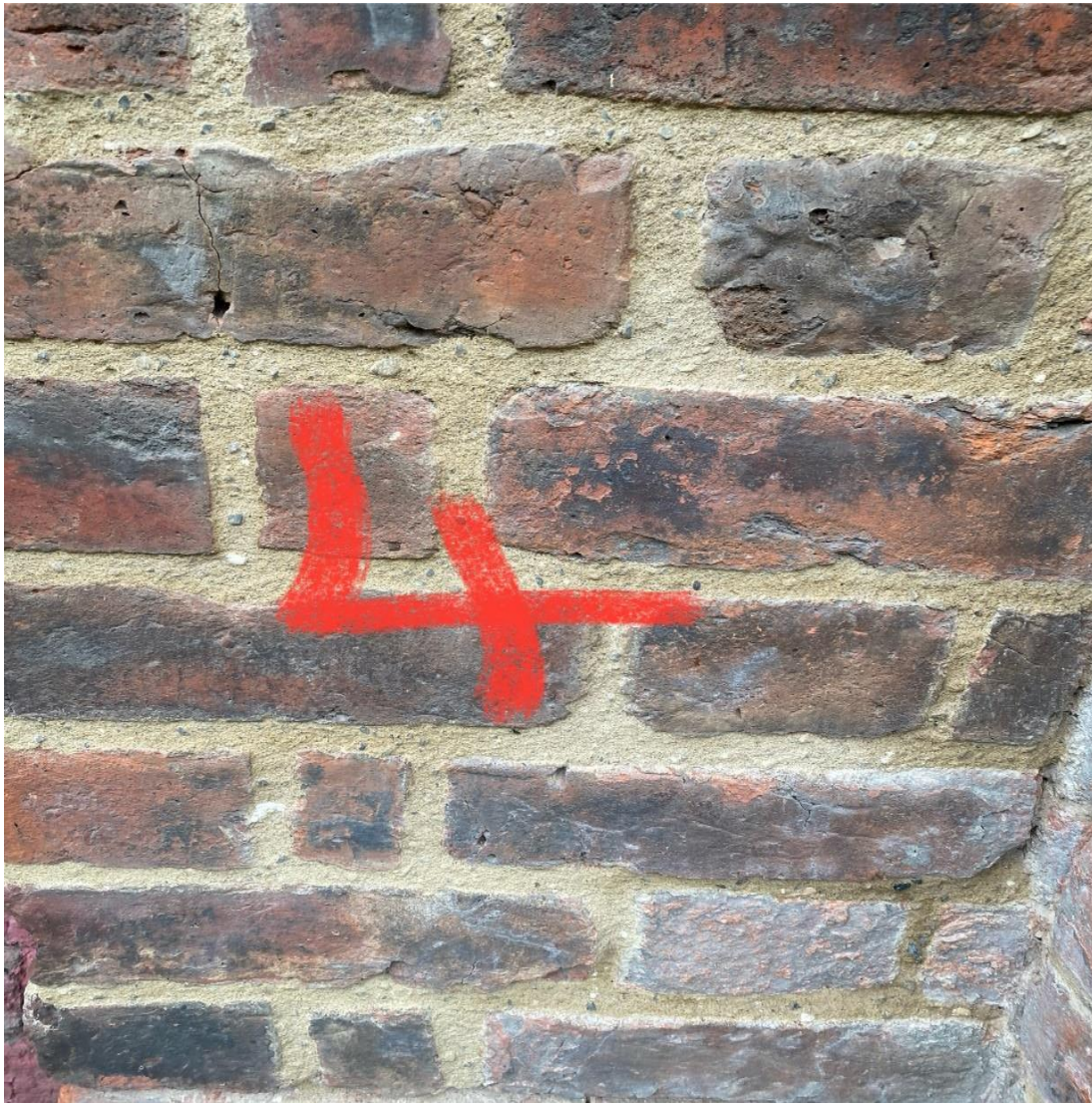
Photo 4. parts 2 Sherbourne 2 parts Leighton Buzzard 1 part NHL 3.5.
