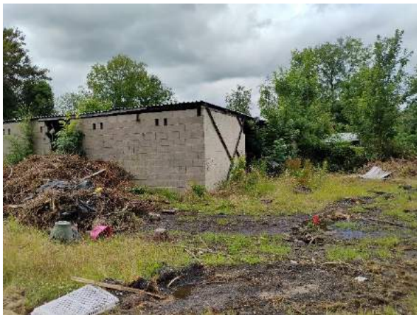
Building 1 – south and east elevations
