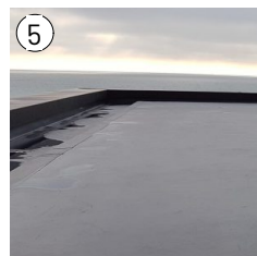
Single ply membrane roof
