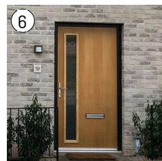
Timber entrance door
