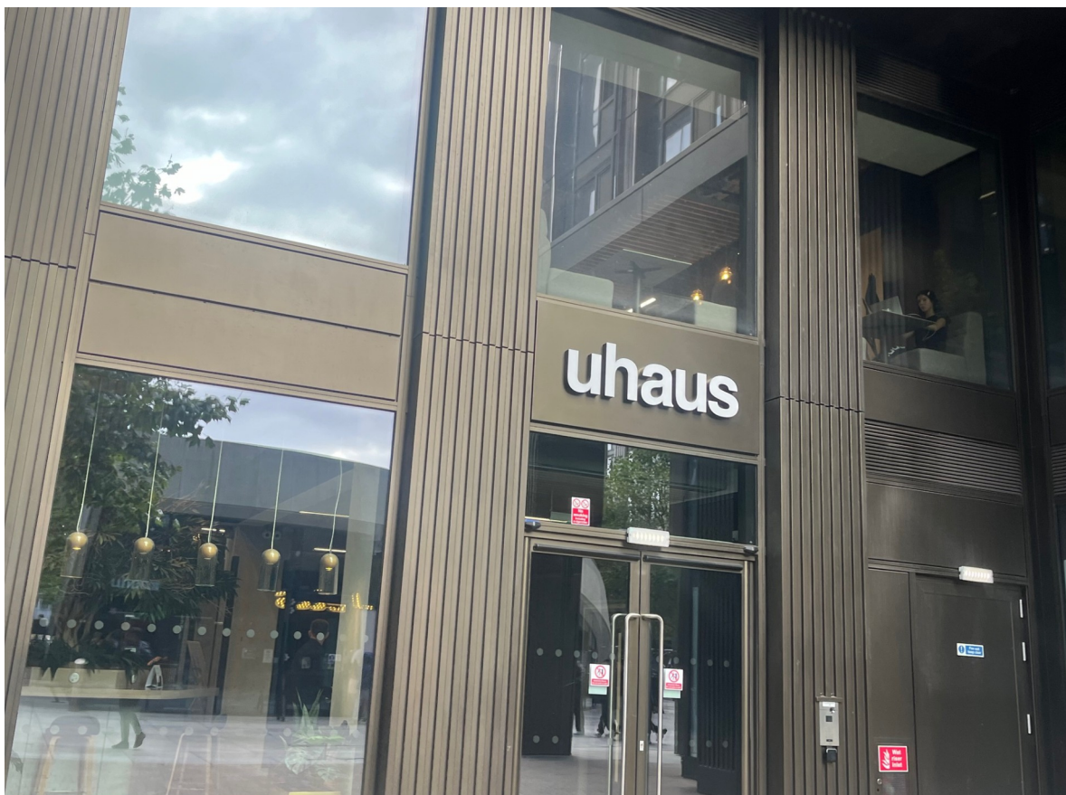
Installed sign to be retained (2)
